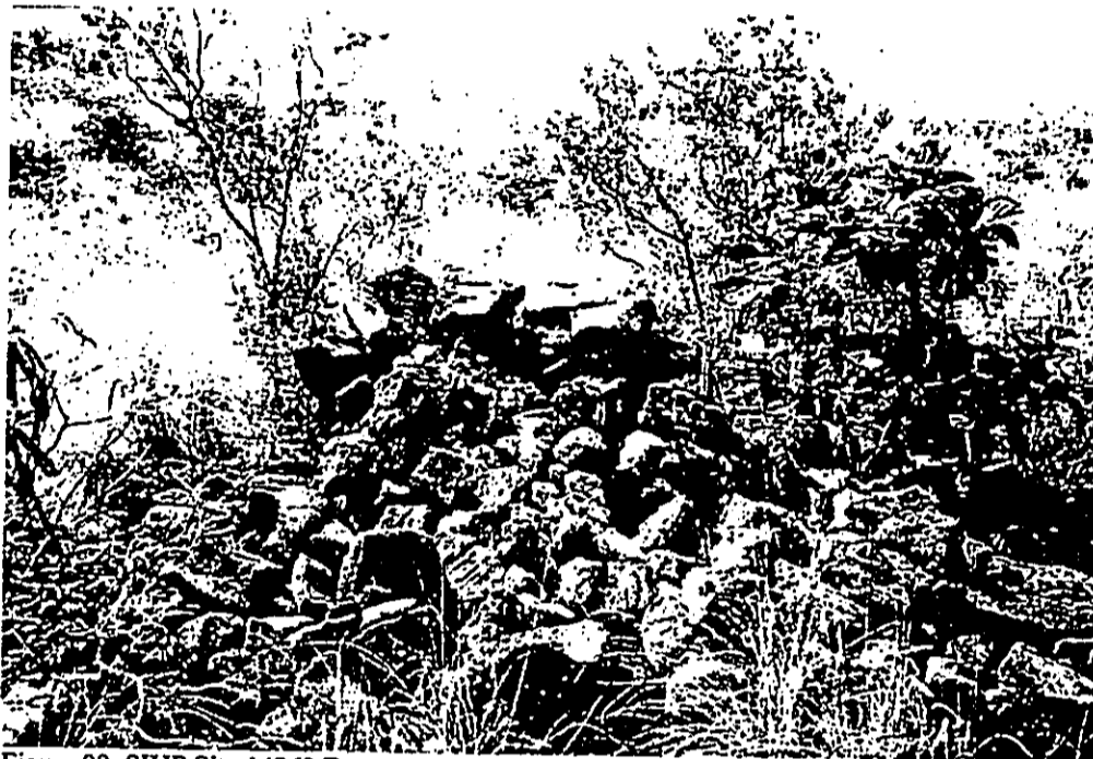
Figure 99. SIHP Site 14362 Feature O view to south of collapsed northern side.
