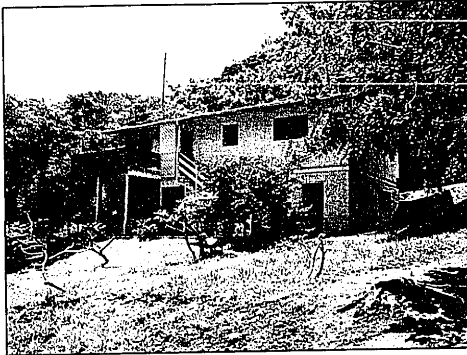
Photograph 1: Former two-story residence presently housing the PCH administrative offices.
