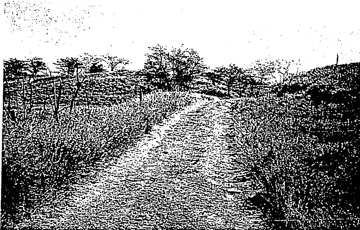
Figure 5. Graded road on study parcel, view to southeast.
