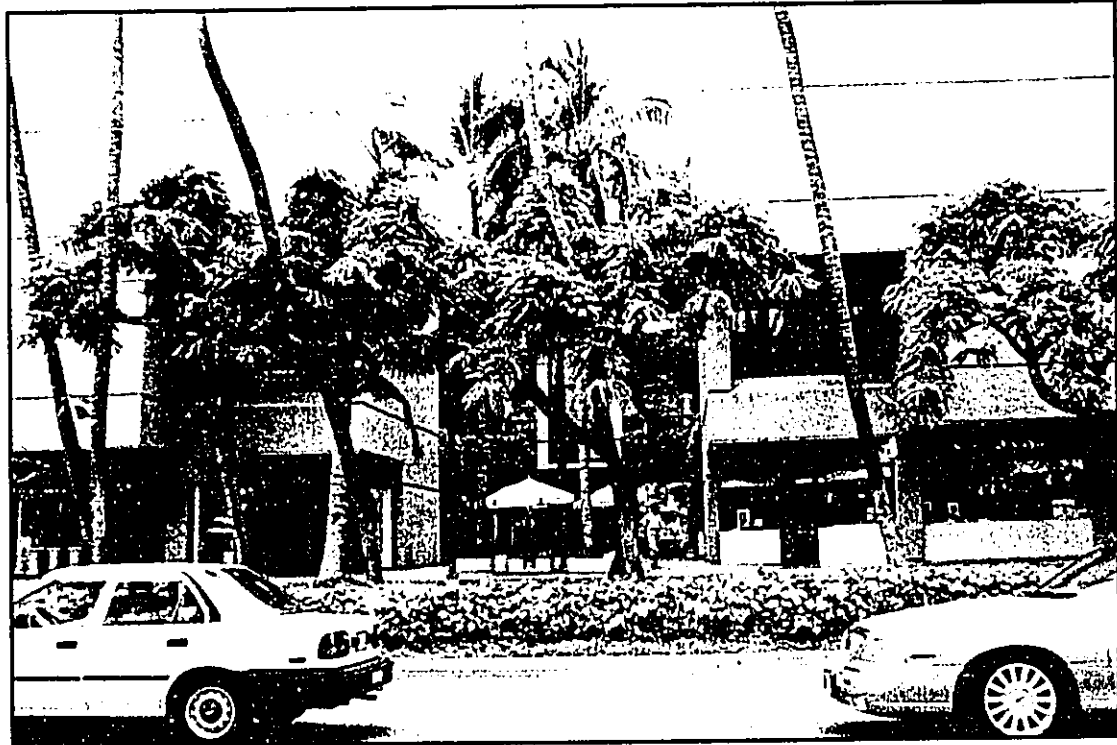
Photograph 10: Entry to Building C Opposite Duke's Lane
