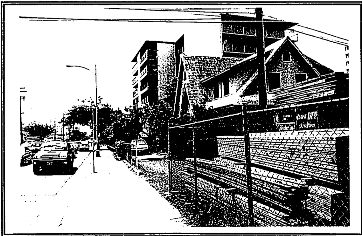
Photograph No. 6 View fronting project looking south on Piikoi Street.
