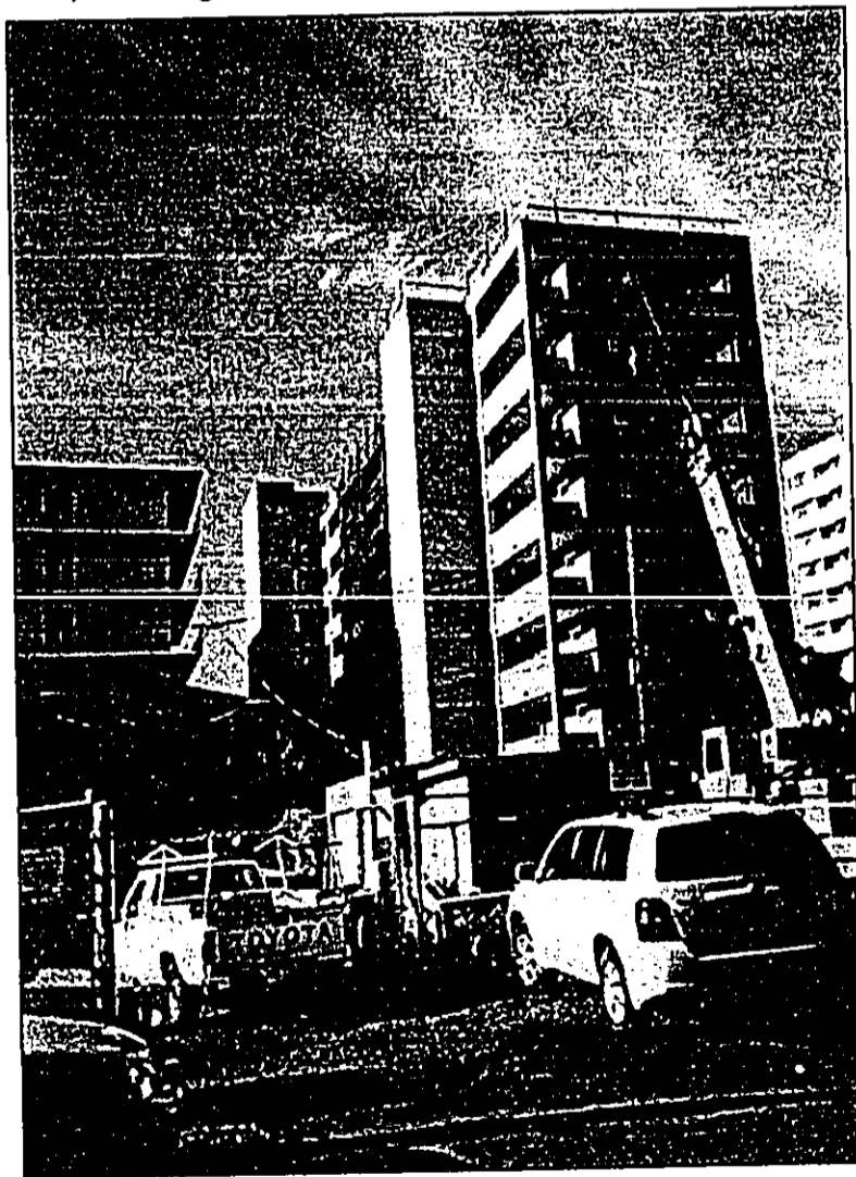
Figure 15. Central section of the project area (behind the chain-link fence), view to the south from Papakū Street
