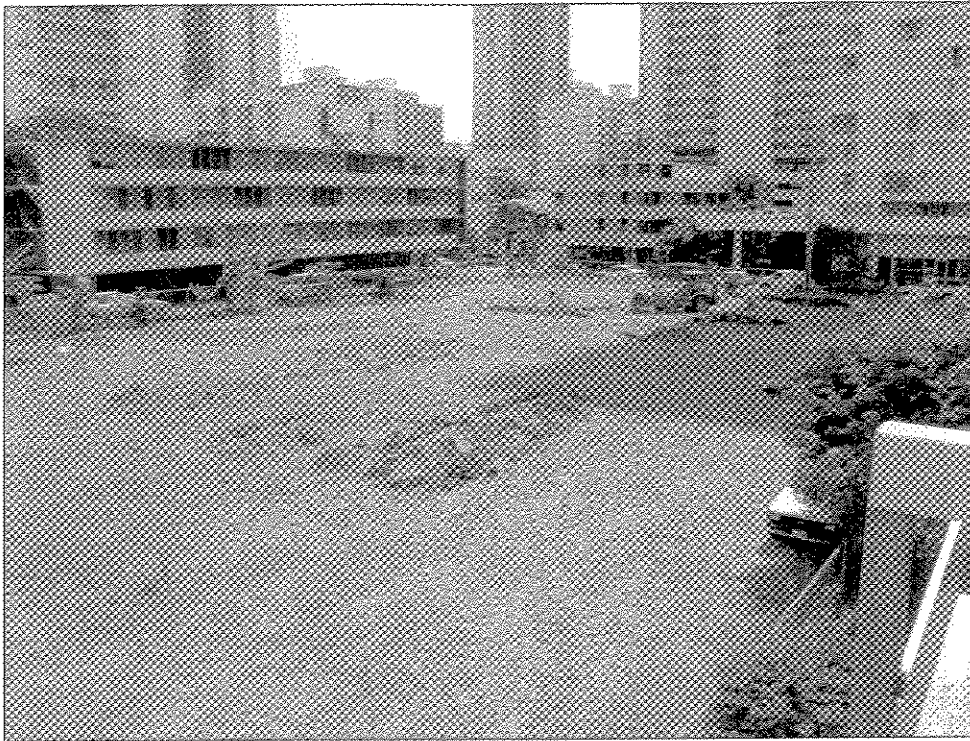
Figure 24. Photograph of project area taken from north corner, view to south
