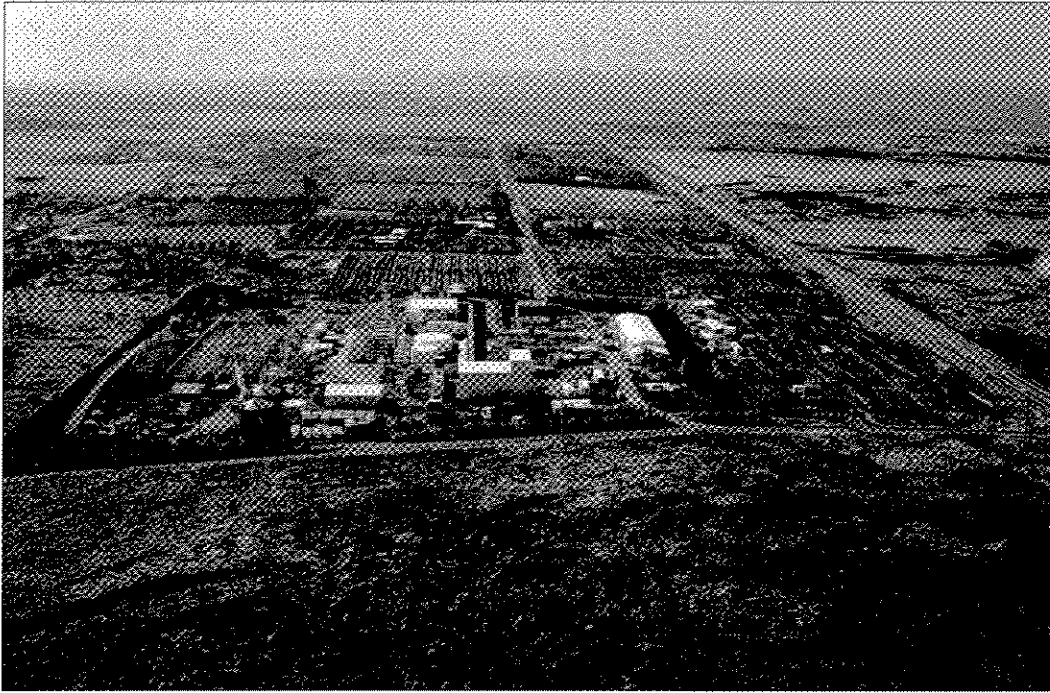
PHOTOGRAPH 3-1: VIEW OF KEAHOLE GENERATING STATION LOOKING SOUTH. THE SECONDARY ACCESS OFF THE RESERVOIR ROAD IS IN THE FOREGROUND.
