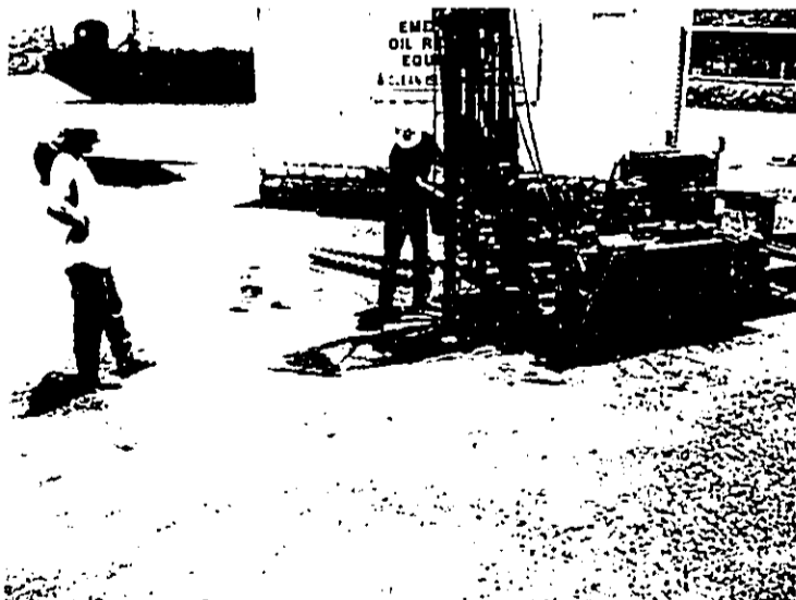
Photo 3. Starting hollow stem auger drilling at SB-1
