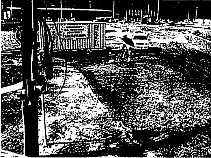
Photo 1. Ground penetrating radar survey at SB-1 location
