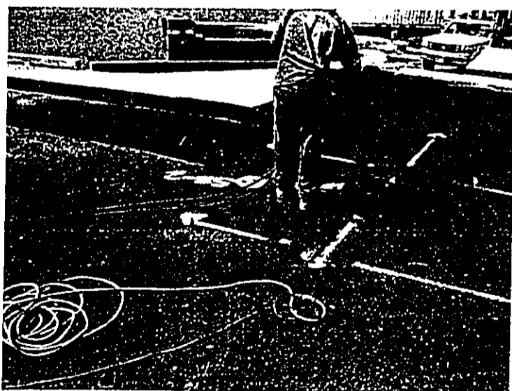
Photo 6. Coring contractor, Pacific Coring, penetrating concrete/asphalt cover material at SB-2
