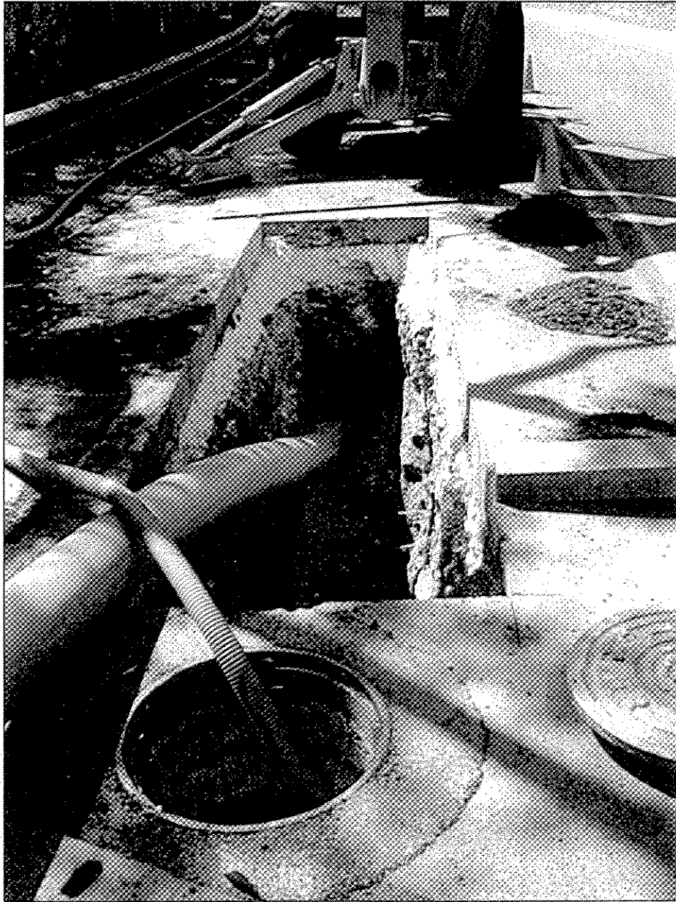
Photo 1: Pipe Bursting Insertion Pit
