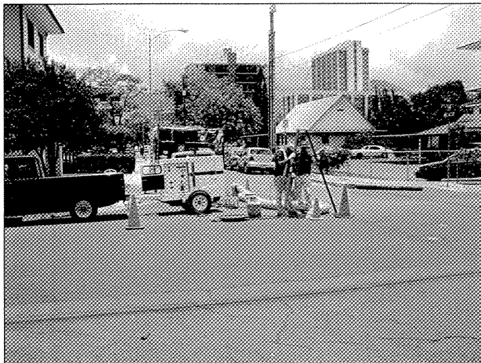
Photo 8: Work area for manhole coating.
