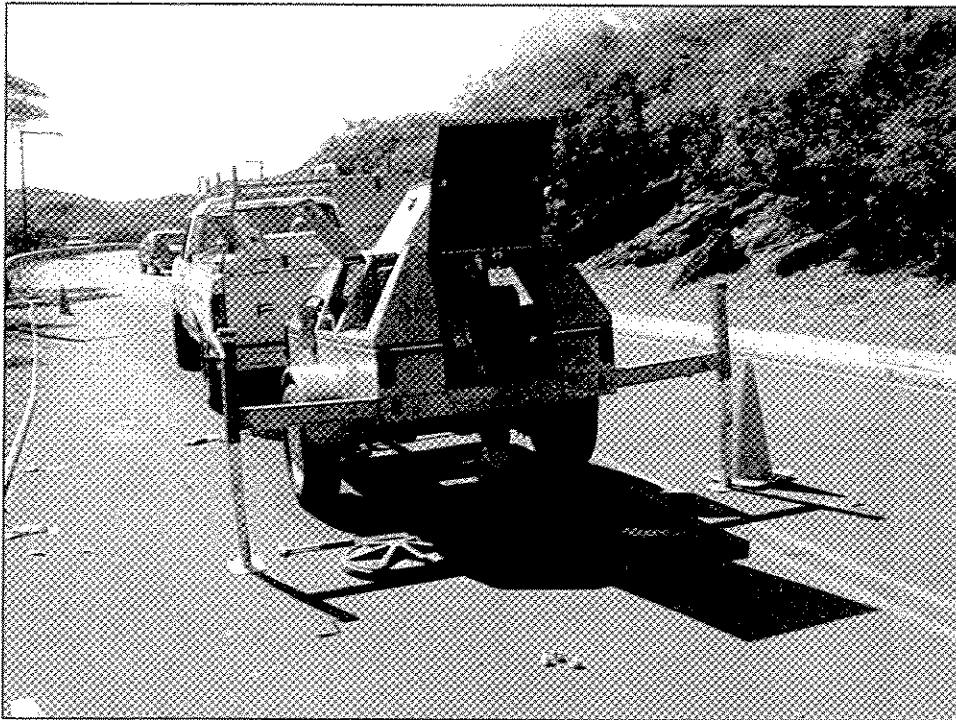
Photo 2: Pipe bursting winch at receiving manhole.
