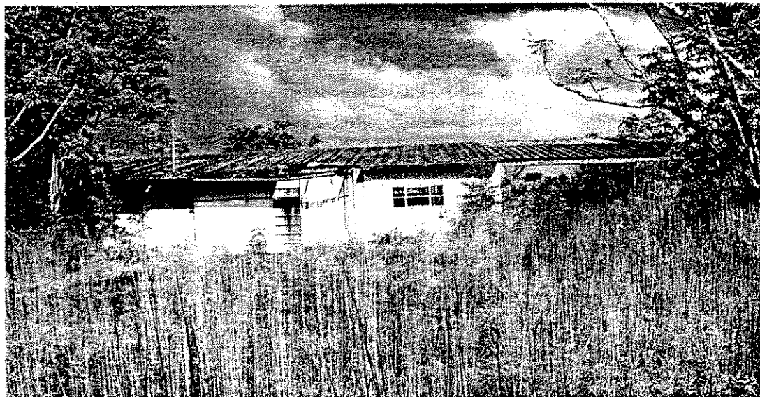
Figure 4. One of several modern building constructed on the study parcel.
