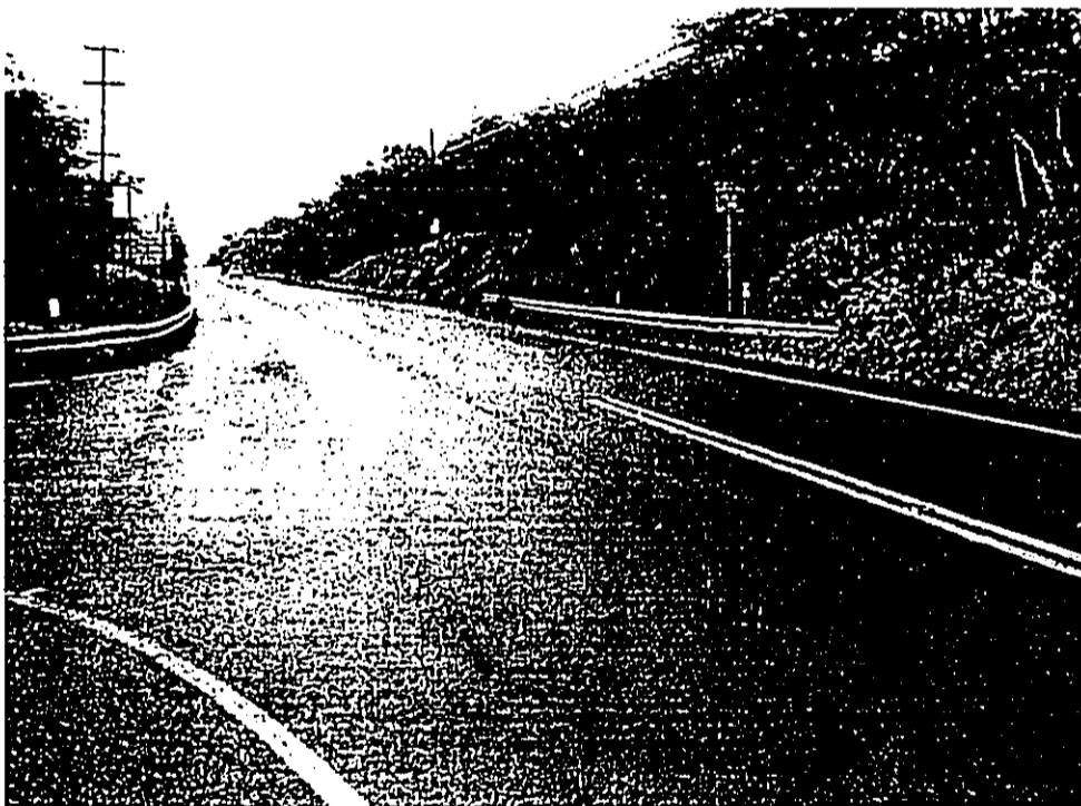
Figure 5 Harbor Access Intersection on Honoapiilani Highway
