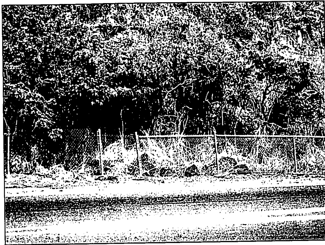
Photo 3: Fallen rocks behind existing chain link fence along Komo Mai Drive.
