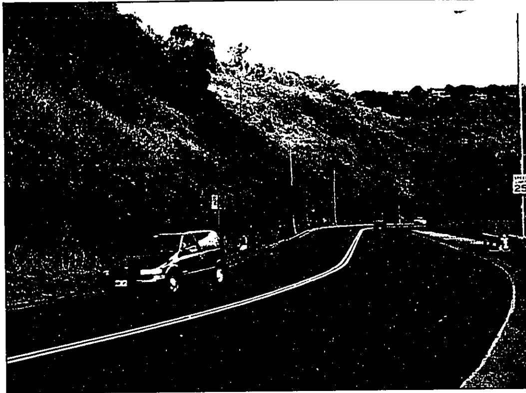
Photo 1: Project area along Komo Mai Drive proposed for installation of mesh and cable net drape systems.
