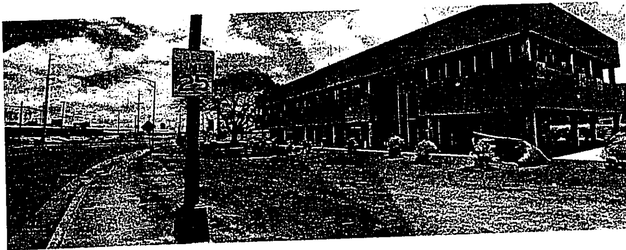
Photo 1: View of Control and Administration Building facing East
