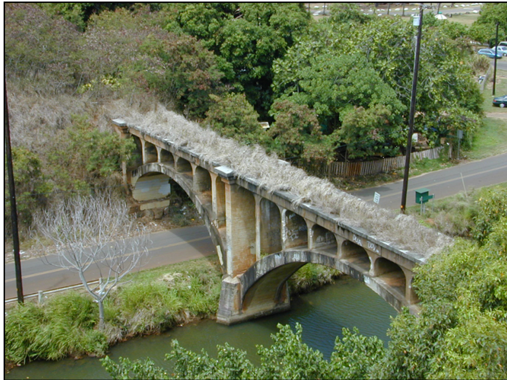
Figure 4a- Photo of the Hanama'ulu Bridge
