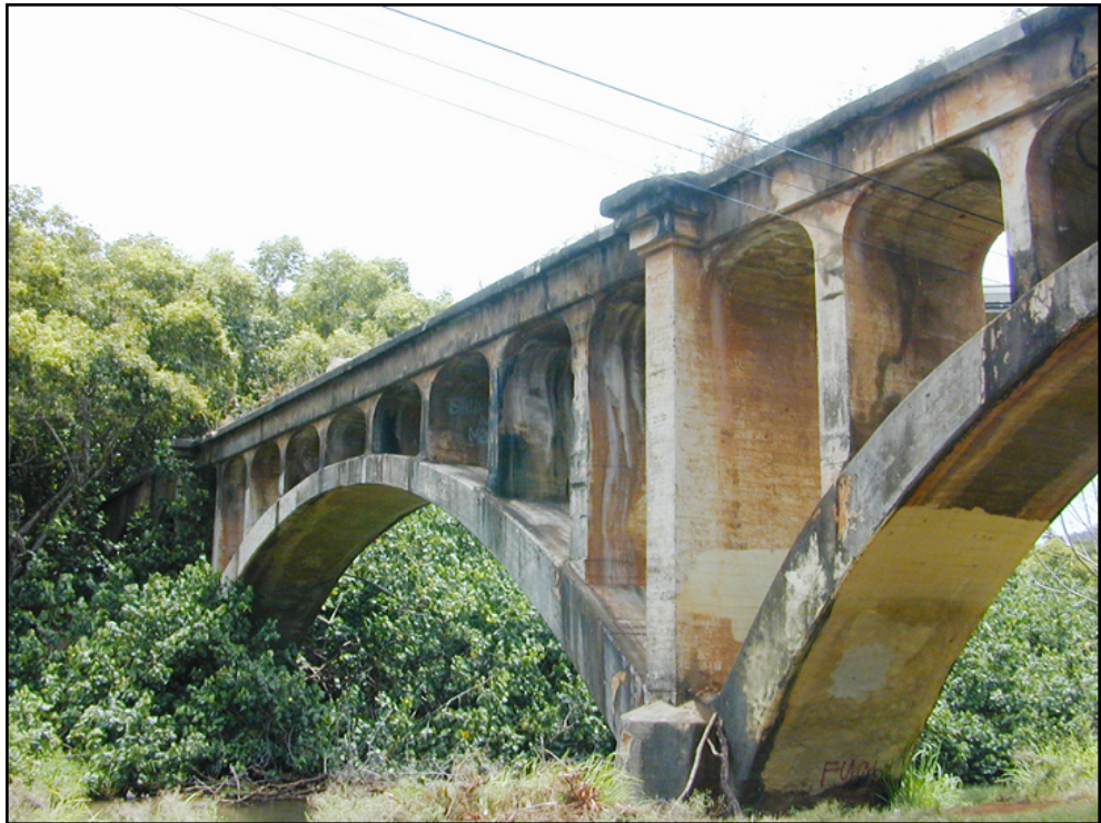
Figure 4b – Photo of the Hanama'ulu Bridge
