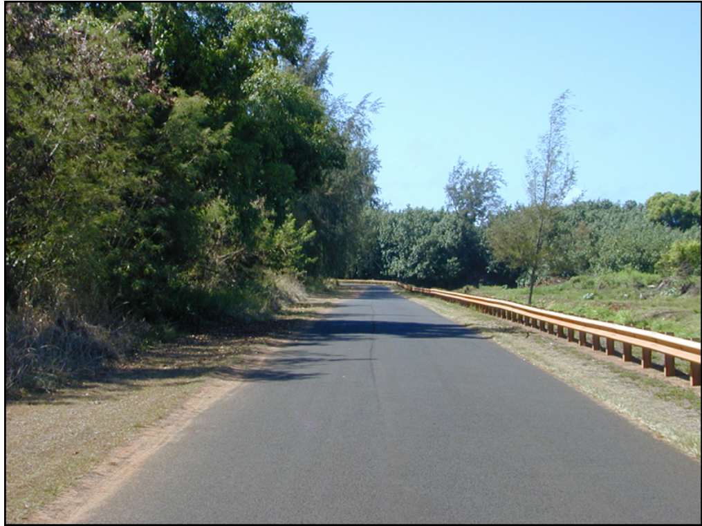
Figure 21b – Photo of Hilton Lane road
