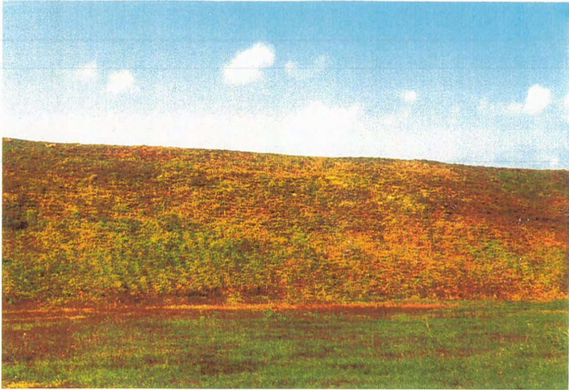
#15 and #16 Proper grading, regrassing and irrigation
