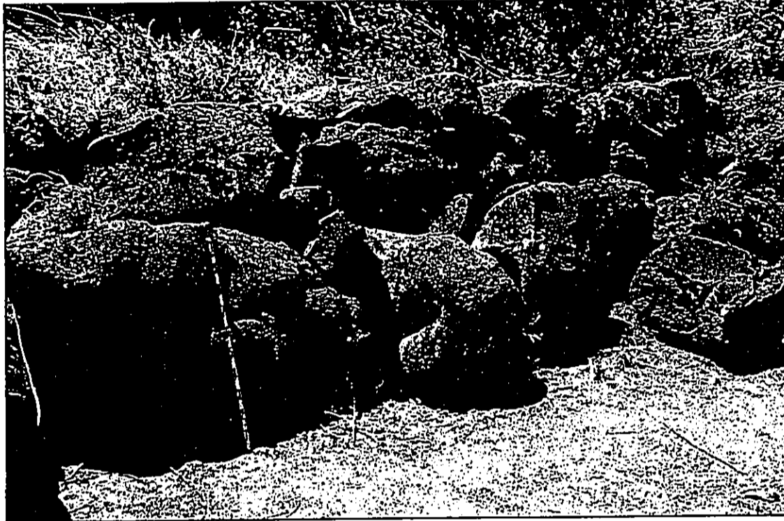
Figure 18. Possible boulder impounding wall on south edge of Alexander Reservoir, view northwest
