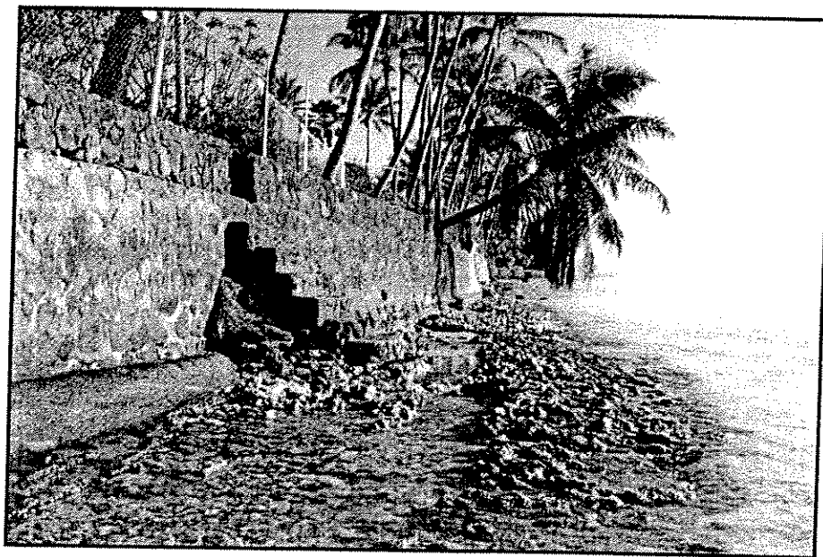
Figure 2-2. View looking east from the project site.
