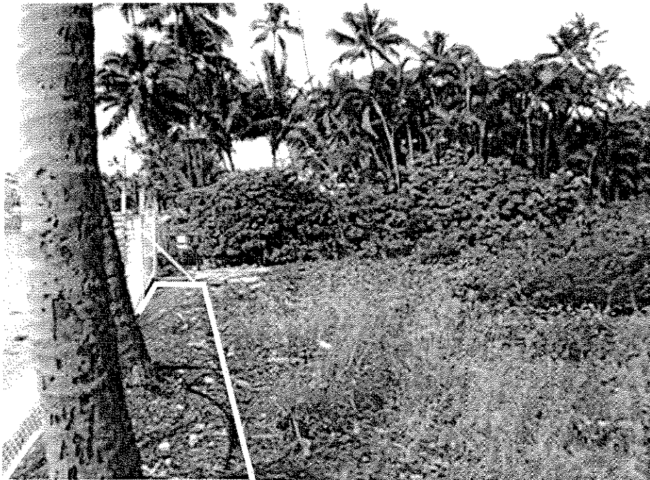
Gravel Fill Behind Seawall: Parcel 10
