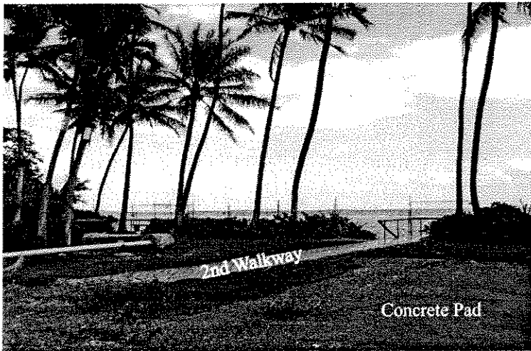
Second Observation Deck, Walkway and Concrete Pad: Parcel 8
