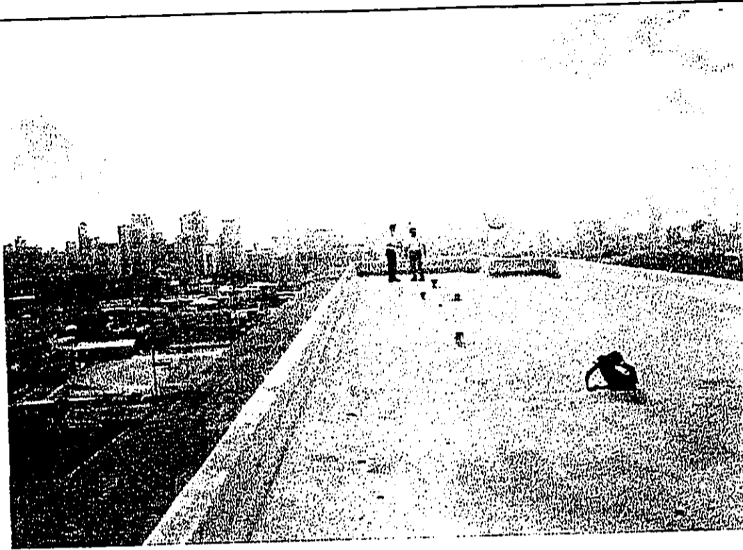
VIEW TO SOUTHERLY END OF ROOFTOP
