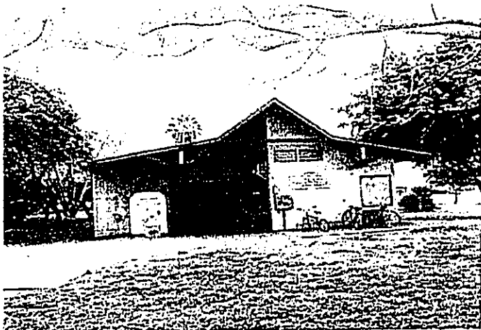
Existing BGCM Clubhse Bldg - Northwest end @ Entry
