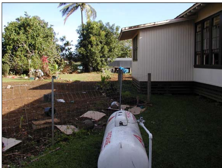
Photo of Cafeteria (Rear) Encroachment Portion
