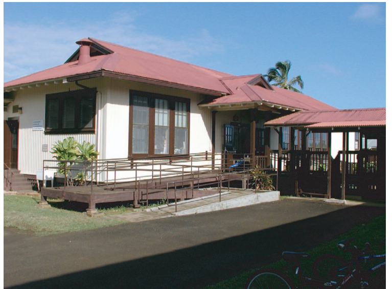
Photo 2 Front View of Cafeteria
