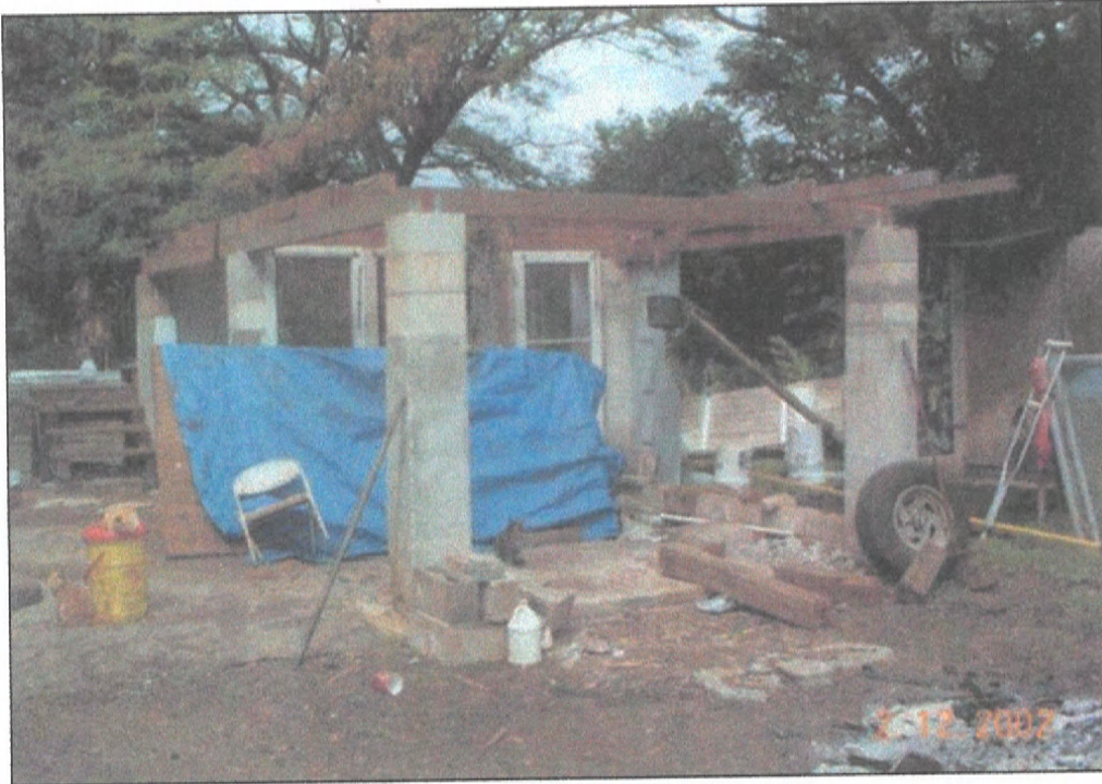
One of the several carports on site prior to demolition.
