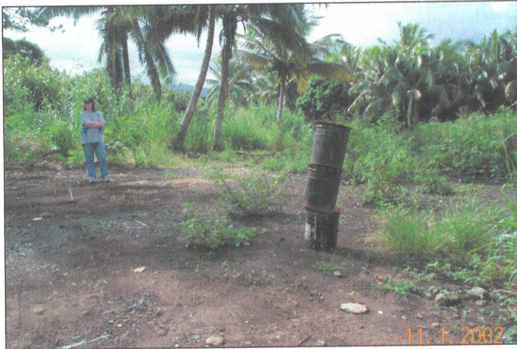
Fig. 3-1, Loc. 5 Remains of the asphalt driveway leading to the three wooden-story buildings and two carports, prior to demolition.
