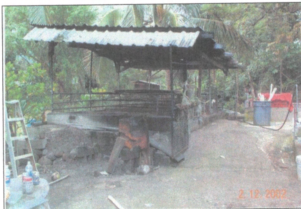
One of the two pig pens on site prior to demolition.
