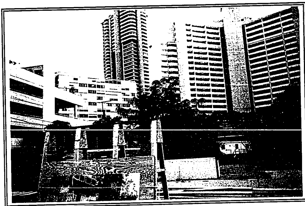
Photograph No. 4 - Photo of the mauka portion of the project site, facing east, showing the temporary office trailer with The Wailana in the background.
