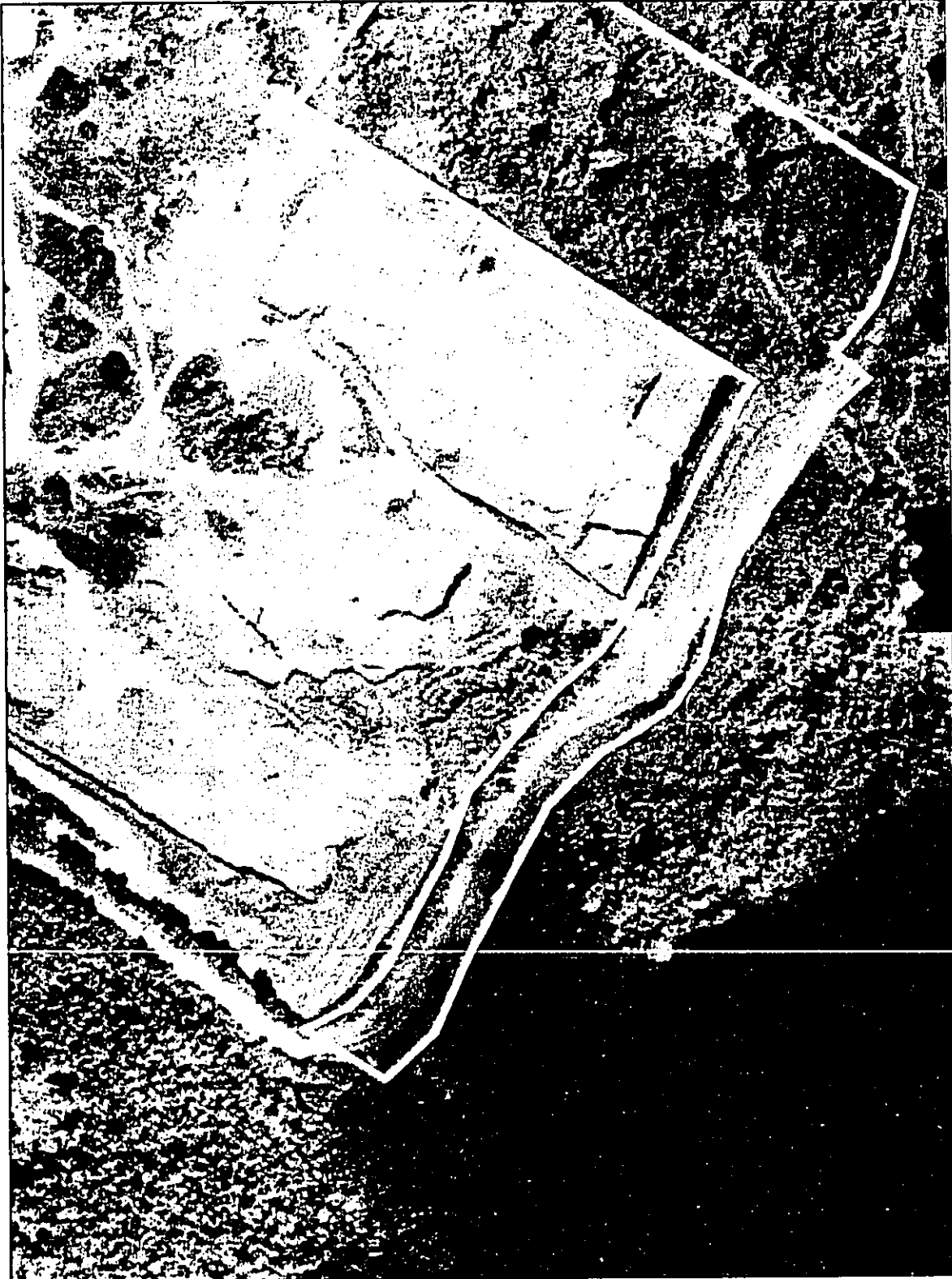
Figure 3. Aerial view of current project area.
