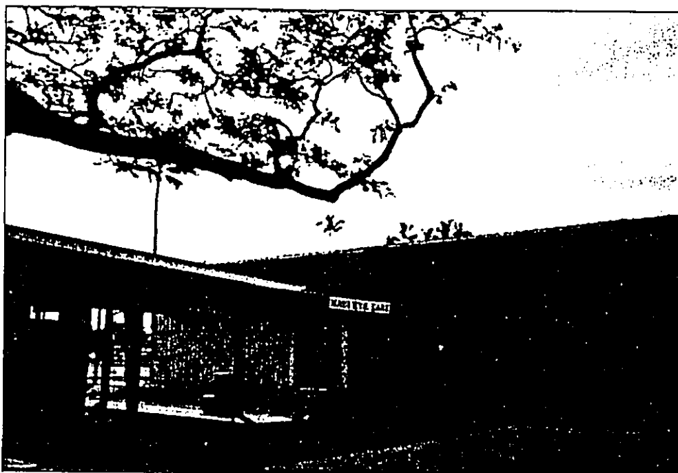
Appendix A Figure 33: Island Dodge/Maui Eye Care, Building No. 31&35. View to Southeast.
