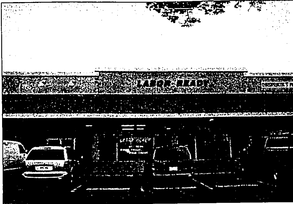
Appendix A Figure 5: Labor Ready, Building No. 3C. View to Southeast.
