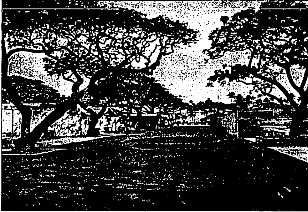
Appendix A Figure 37: Project Area Overview (looking down Mall). View to Northwest.
