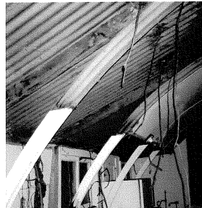
Quonset hut interior framing. Note the existing 2" X 4" steel framing with wood framing.
