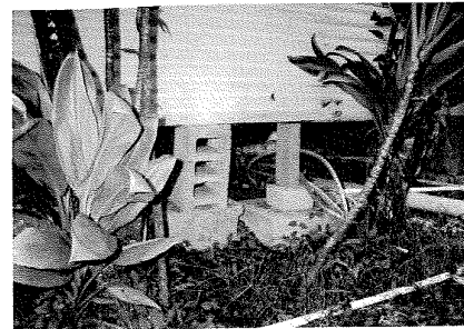
Quonset Hut Typical Foundation Post and Pier. Note due to severe rusting concrete masonry is being used to support steel girders.
