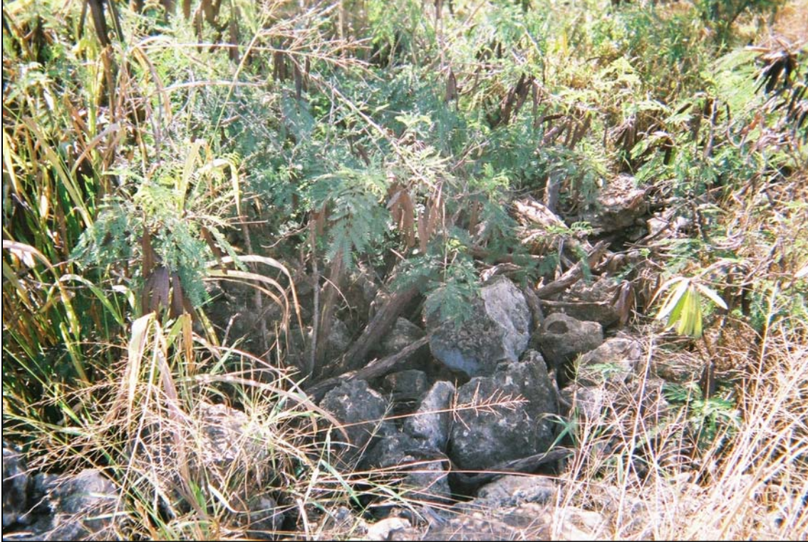
Figure 6. Rubble filled sinkhole (1 x 1.5 m).
