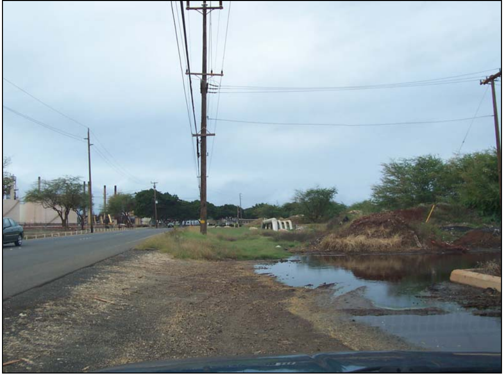
Figure 9. Proposed pipeline easement along Malakole Road (view to W).
