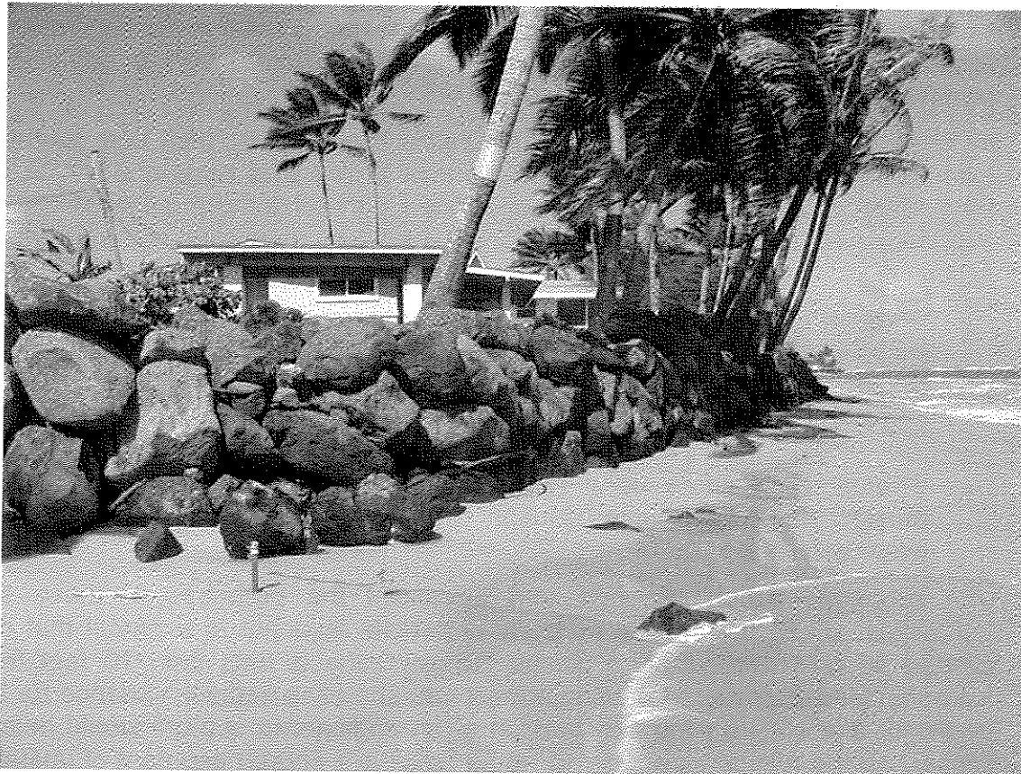
B. December 3, 2004 the existing illegal temporary seawall that is beginning to come apart at the corner. The vertical pipe represents the corner of the parcel. At high tide
