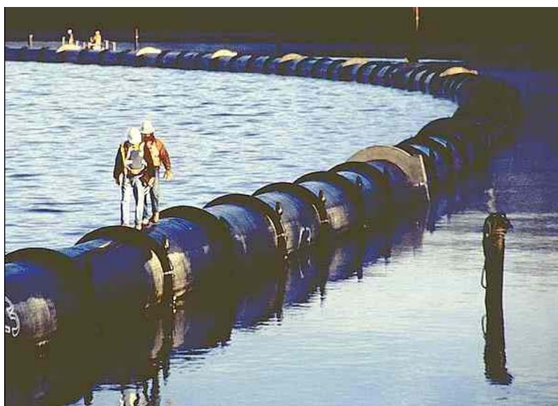
Figure 2-6: A 63-inch Pipeline with Ductile Iron Stiffeners (Source: MOE, 2005a)
