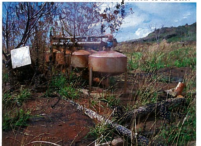
Photo 6: Old irrigation pump system located near the northwestern corner of the Site.
