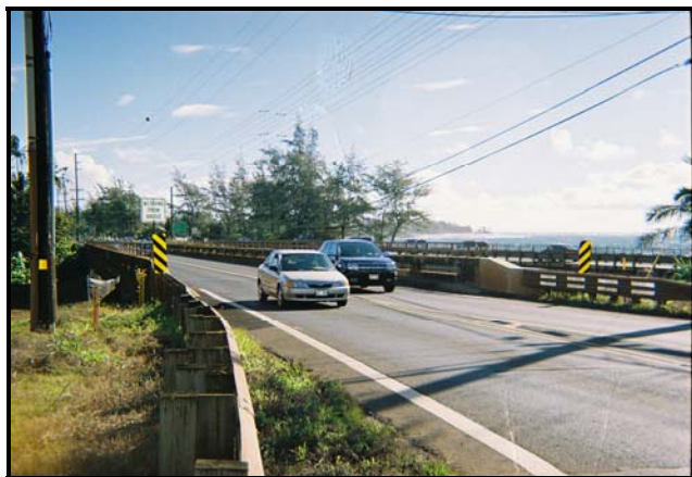
Looking North on Kuhio Highway near Wailua River
