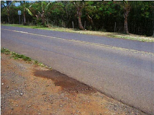
Photo 8: Stained soil observed along the edge of Leho Drive in front of the KIUC electric substation.
