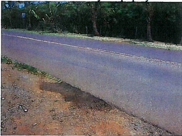
Photo 8: Stained soil observed along the edge of Leho Drive in front of the KIUC electric substation.
