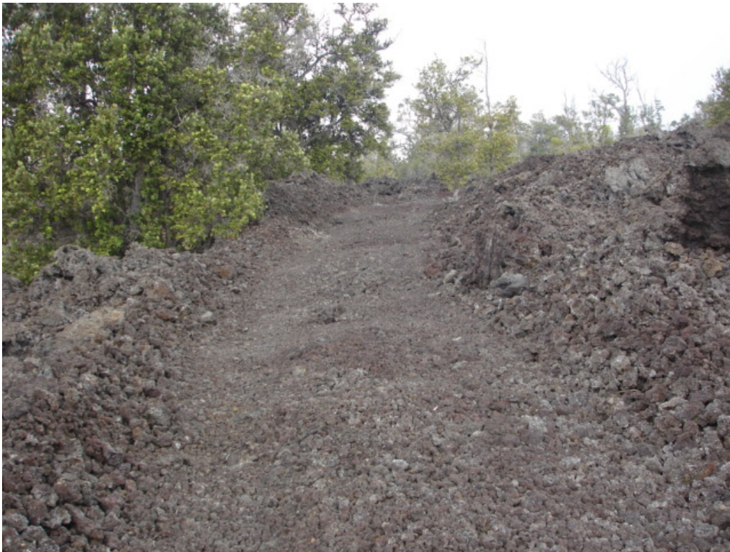
Figure 5. Bulldozed road coursing through the central portion of the study parcel.
