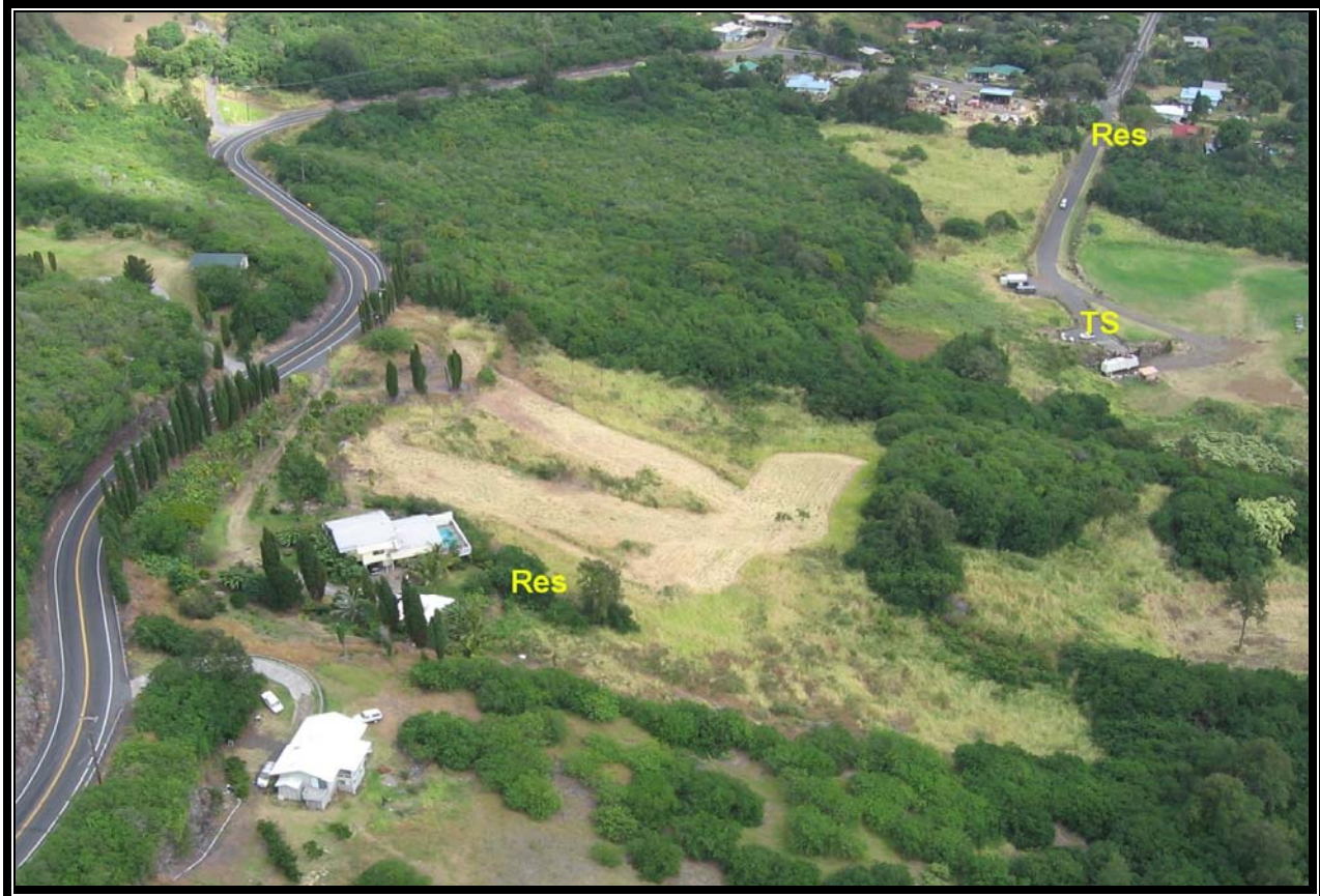
Figure 4-1 Convenience Centers in Residential Areas (Page 3) Wai'ohinu – Several homes within 500 feet, more within 800 feet
