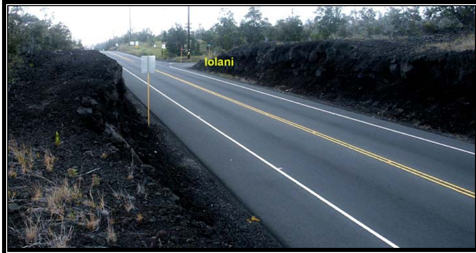
Figure 4-5. Views Along Highway View from Near Road A to West
