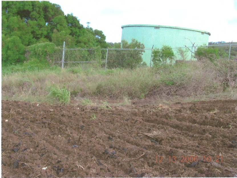
North View of Existing Well Storage Tank
