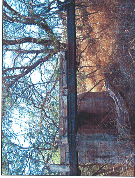
Figure 21. Bridge bed component of Feature B showing support beams and flume construction, view to west
