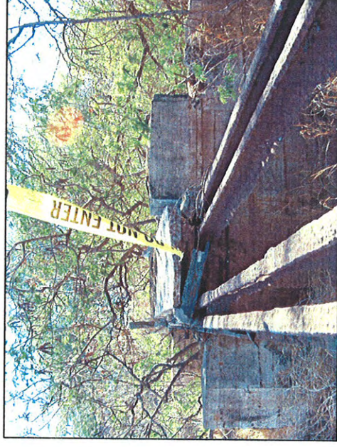
Figure 21. Bridge bed component of Feature B showing support beams and flume construction, view to west
