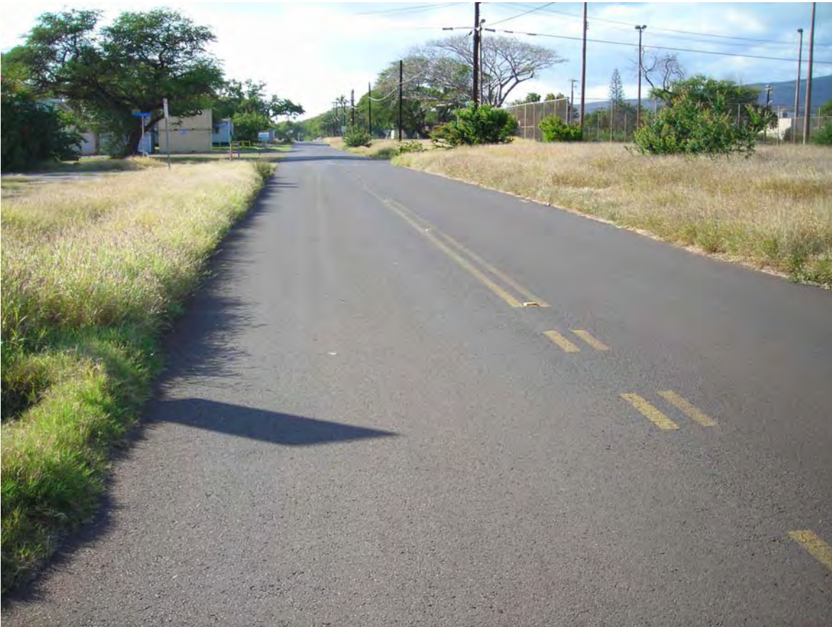
Exhibit III-15: View of Yorktown Road
