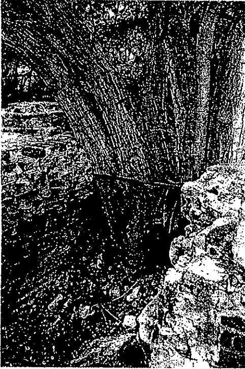
Photo 20 - Large tree growing within the brick structure.
