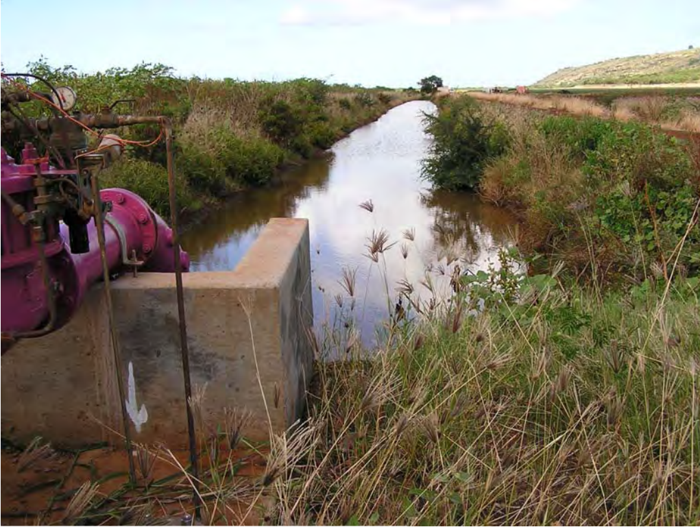
Figure 1. Effluent Isolation Ditch
