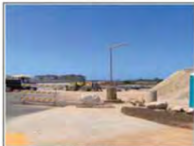
Photo 2B Project Site entrance from Kapolei Parkway facing SW
