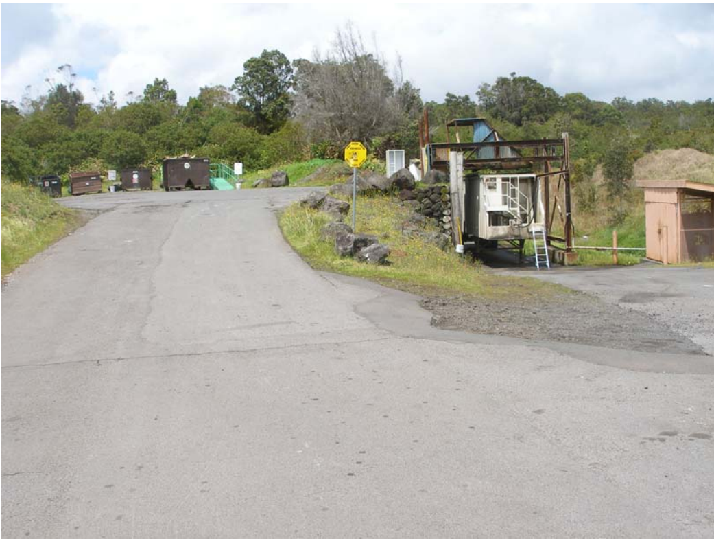
Figure 4. Volcano Transfer Station, view to the southwest.
