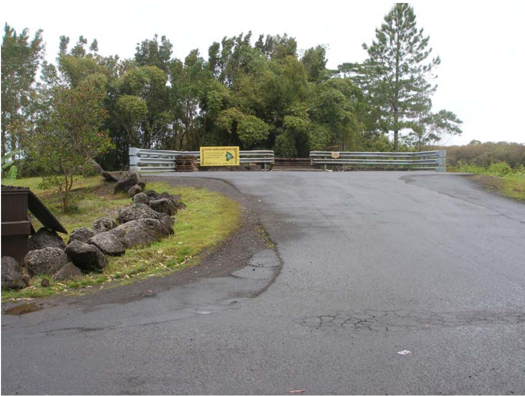
Figure 4. Glenwood Transfer Station, view to the east.
