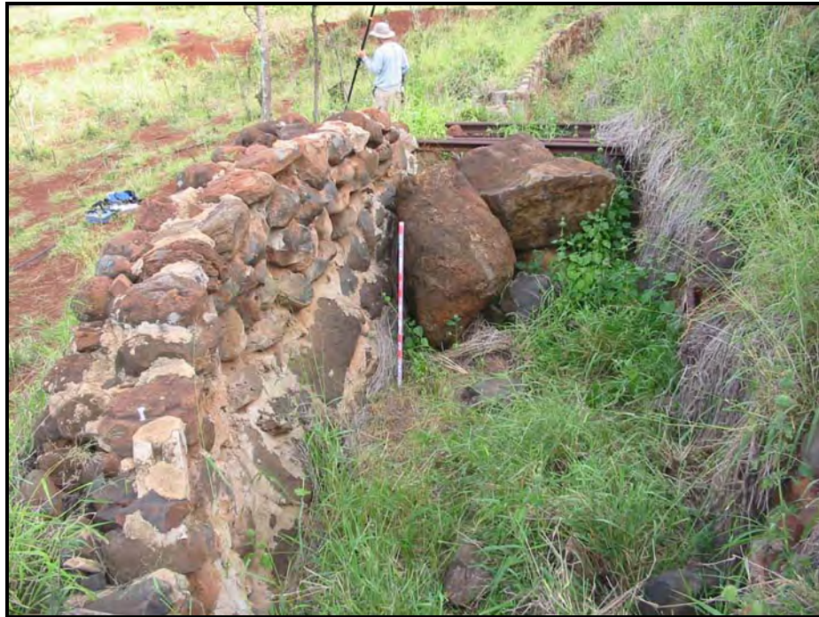
Figure 35. South view of length of reservoir ditch
