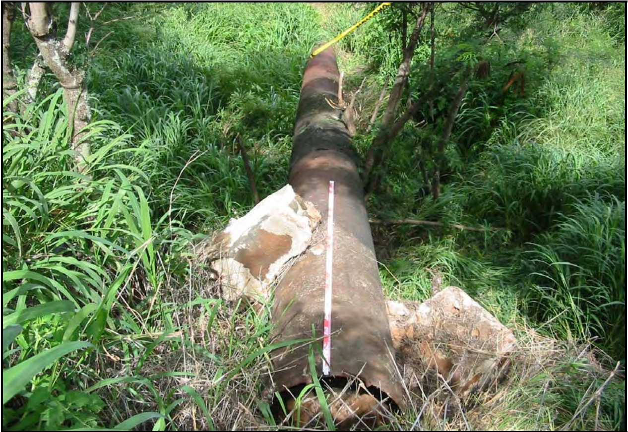
Figure 22. North view of 20-inch iron pipe, Feature A, SIHP No. 50-80-12-6950.
