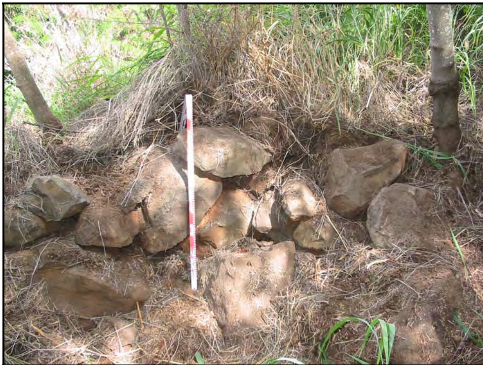
Figure 27 East view of Retaining Wall 1.
