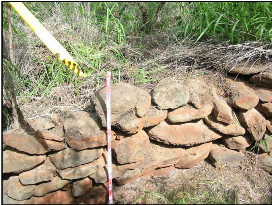
Figure 31. NE view of Retaining Wall 3.
