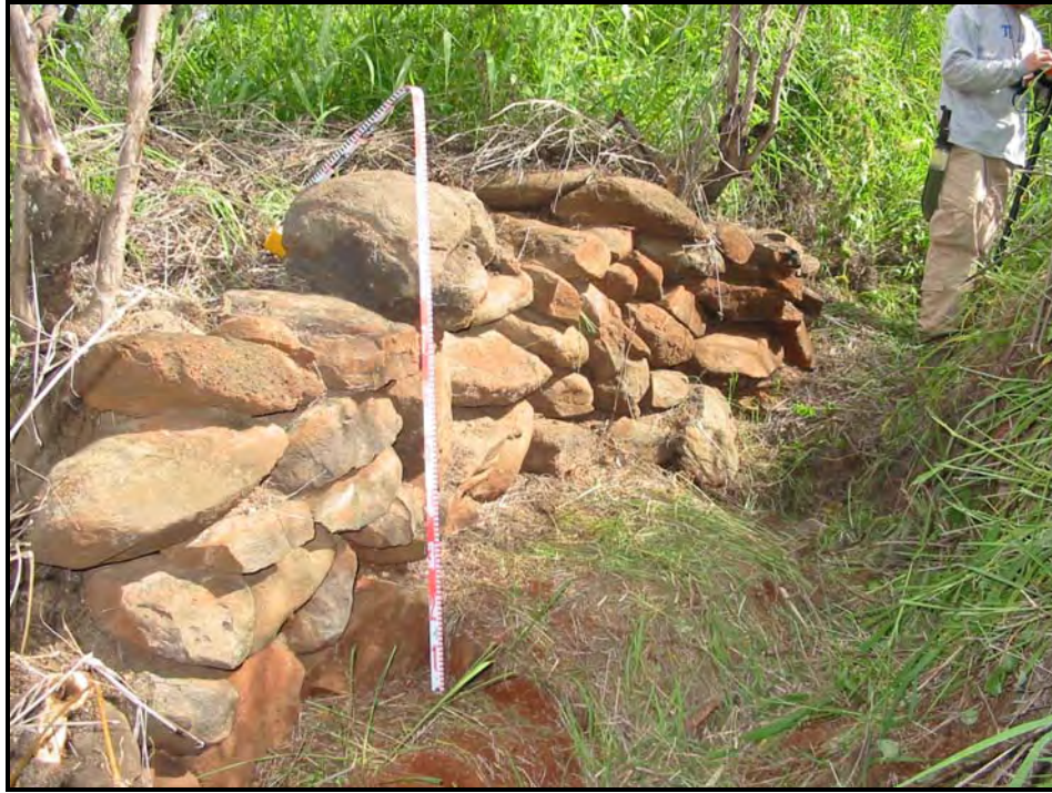
Figure 30. East view of Retaining Wall 3, showing curve to the south, upslope.
