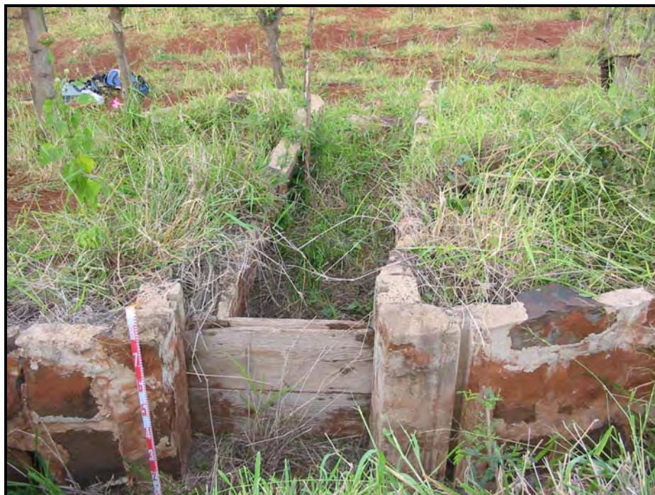
Figure 36. East view of central outflow ditch and gate
