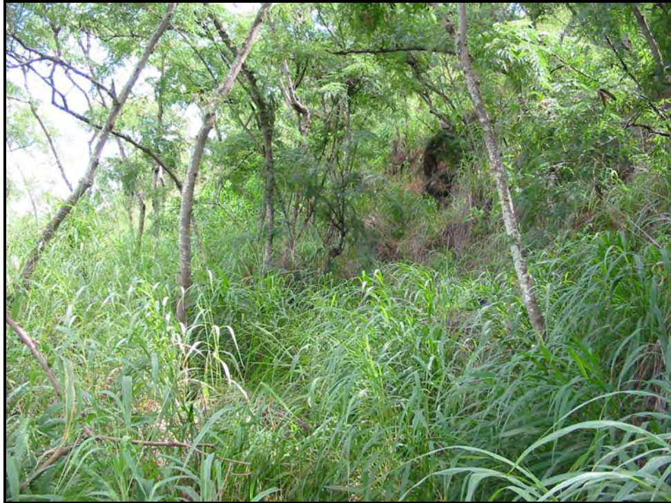
Figure 28 East view of ditch, between Retaining Wall 1 and Retaining Wall 2.
