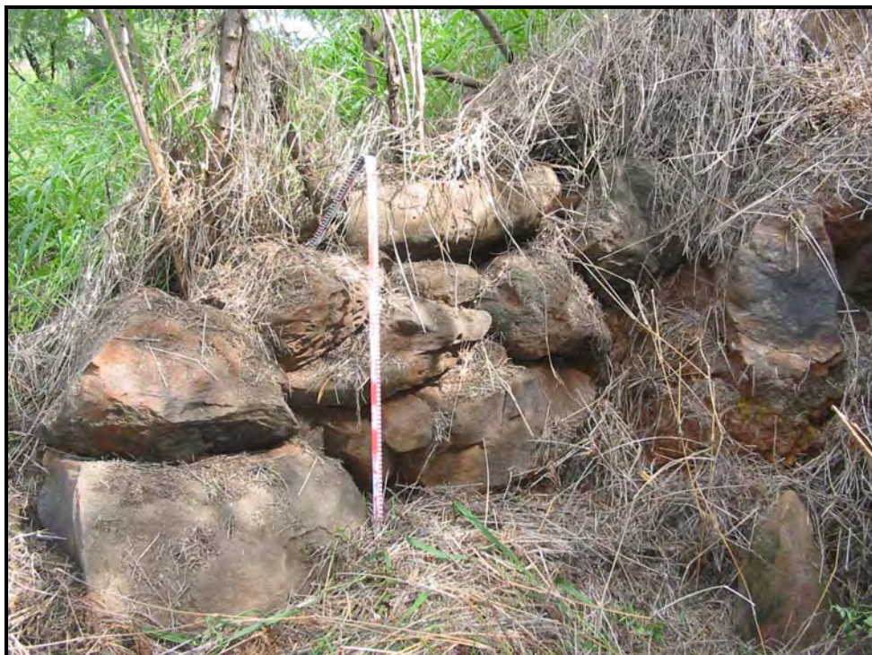
Figure 29 NE view of Retaining Wall 2.
