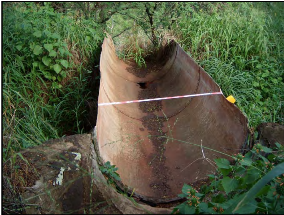
Figure 43. North view of metal flume, Feature A, Site -2268
