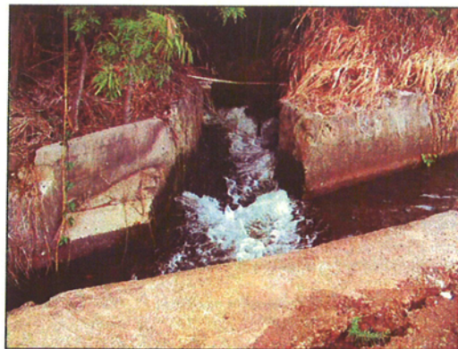
Figure 15: Site 50-50-04-5729 Ditch (at center) flowing into Waihee Ditch (50-50-04-5197). View to West.
