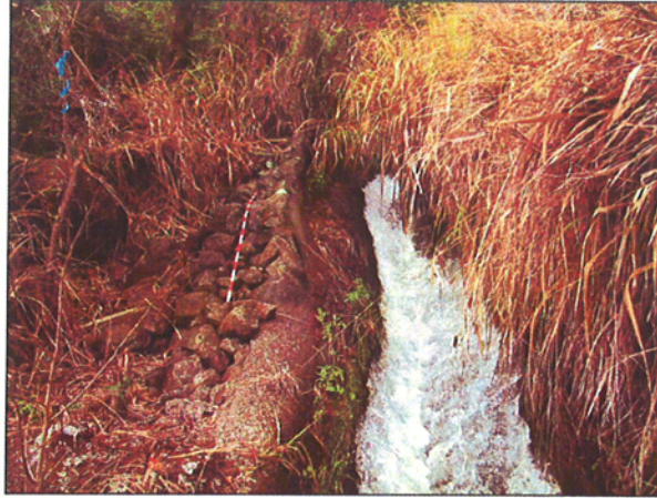
Figure 13: Site 50-50-04-5729 Ditch. View to West.
