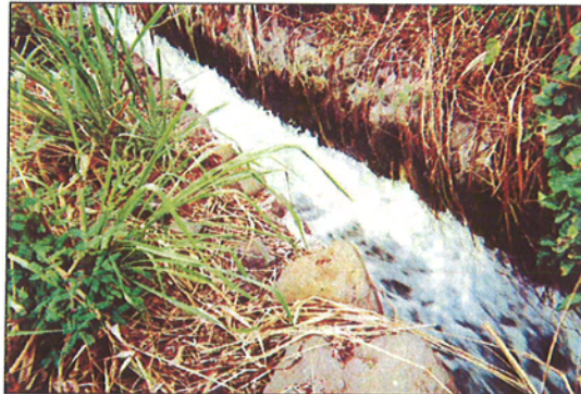
Figure 14: Site 50-50-04-5729 Ditch, Showing Rock and Mortar Construction of Side Walls. View to Northwest.
