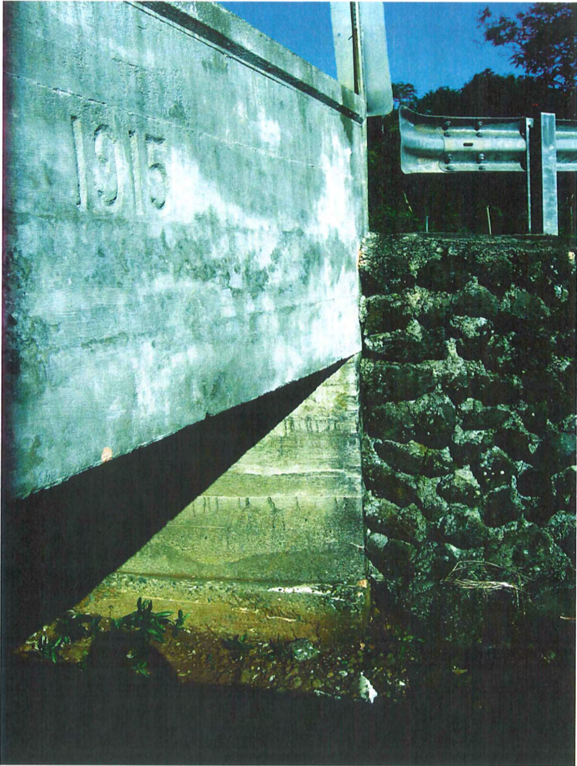
Figure 7: View to North of the Culvert Abutting the Bridge
