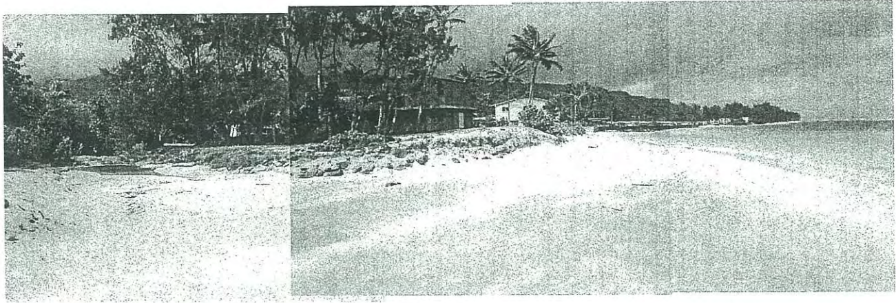
View westward from stream mouth. Note eroded condition of embankment on west side of the stream. Continuous line of seawalls protect entire central shore frontage within the embayment.
