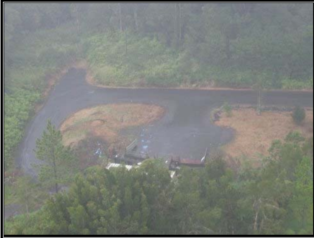
Figure 3a Photographs of Glenwood Convenience Center
