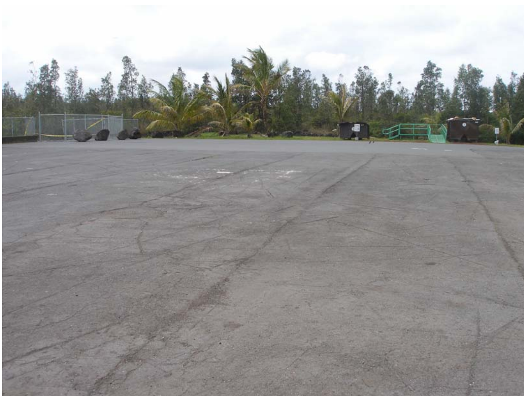
Figure 5. Pāhoa Transfer Station asphalt paved surface, view to the northwest.
