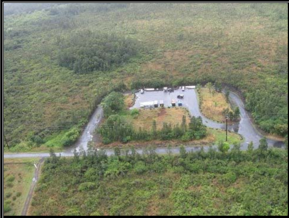
Figure 3b Photographs of Pahoa Convenience Center
