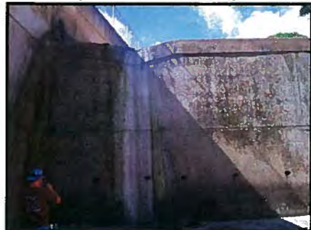
Drop structure; note lack of water and sheer drop that prevents migration.
