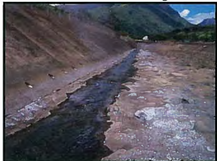
Concrete-lined low-flow stream channel upstream from water diversion structure.
