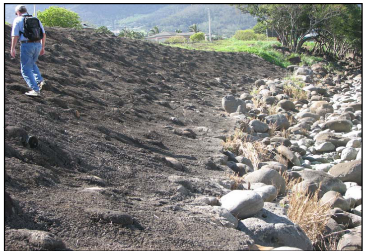
Maintenance performed by Maui County includes placing stone along the toe of the levee as an interim repair measure
