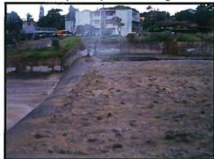
Smaller drop structure, with water diversion feature in the background.
