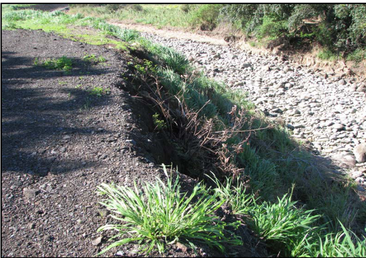
Slope failure of levee on right bank at approximate Station 39+00
