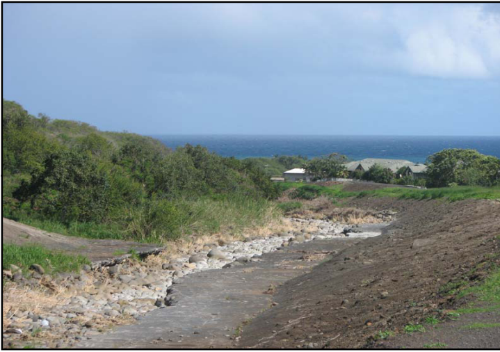
View looking at the area of "boulder concrete" that is being undermined by erosion
