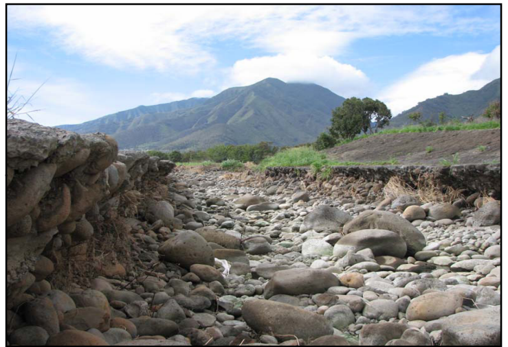
Channel invert eroded 6' to 8' below original channel cutoff walls
