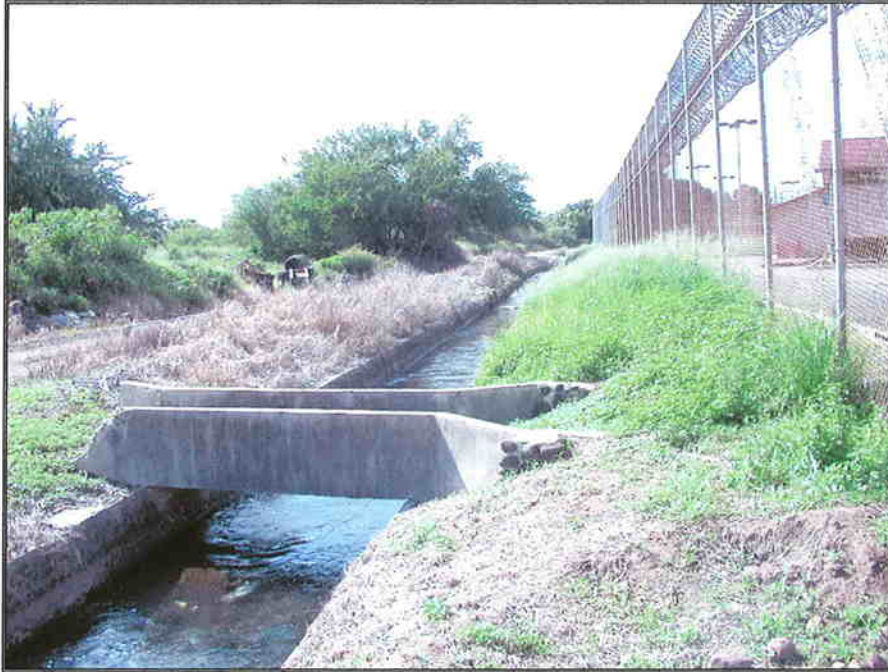
Photograph 3: General view to the southeast along section of Spreckels Ditch. HC & S Co. access road is at left, project area is to left of road.
