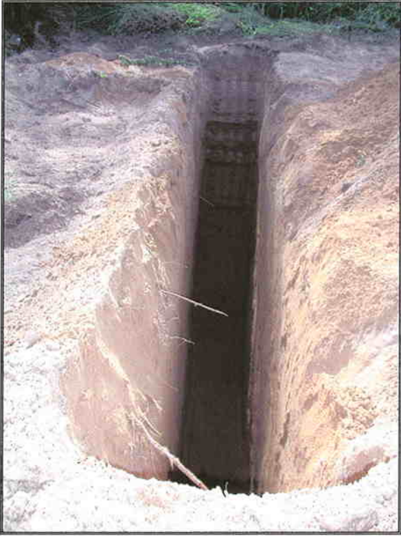
Photograph 10: View to the northeast of BT 7.
