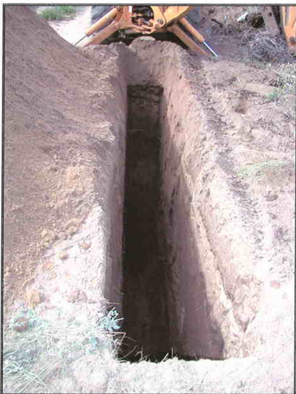
Photograph 6: View to the northeast of BT 2.
