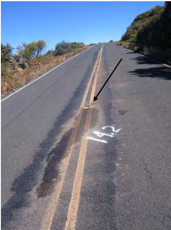
Photo #5 & 6---Segment 2, MP 14.2 & 12.1, Typical pavement distress along centerline of roadway, Note: water flowing through cracks and pavement staining due to migration of fines.
