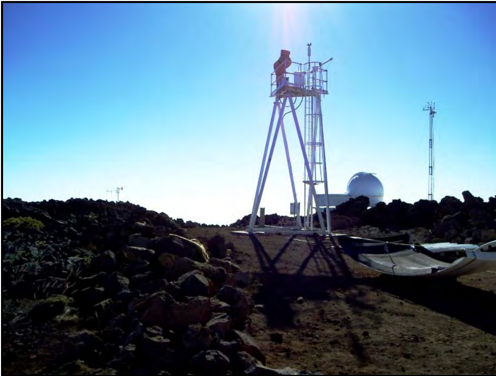
Photograph 4: View to the southwest of the data tower and weather tower (right), note push pile at left and construction materials at right; Mees Observatory is in the background.
