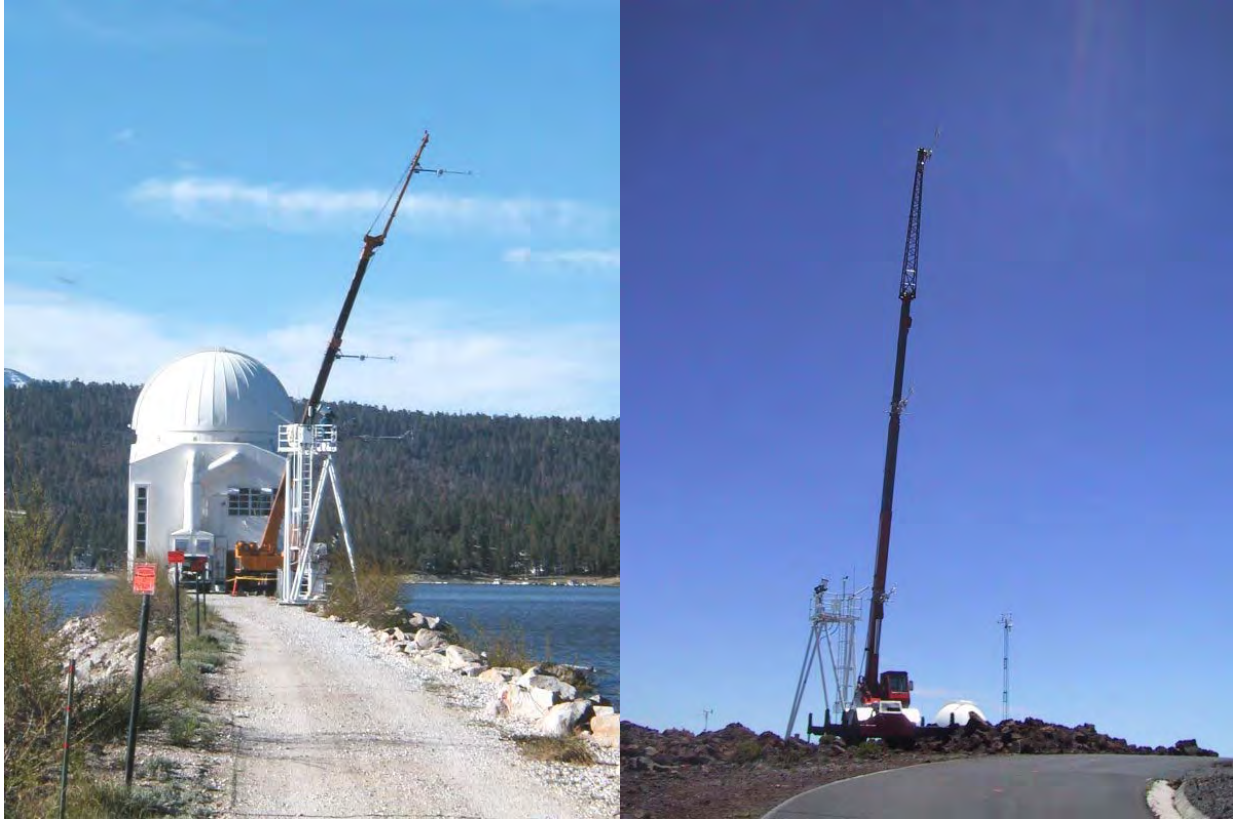
Figure 9.8: The in-situ C_n^2 measurements underway at Big Bear (left) and Haleakala (right).
