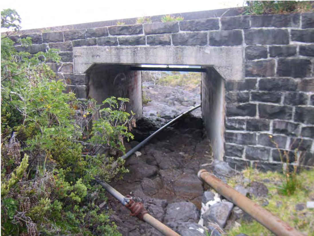
Photos 14, 15 & 16-----Typical open bottom Concrete Box Culverts with Masonry hdwls.
