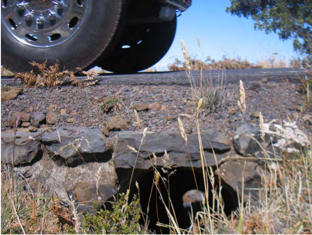
Photo #18 ---Typical metal culvert with masonry headwall and note minimum cover
