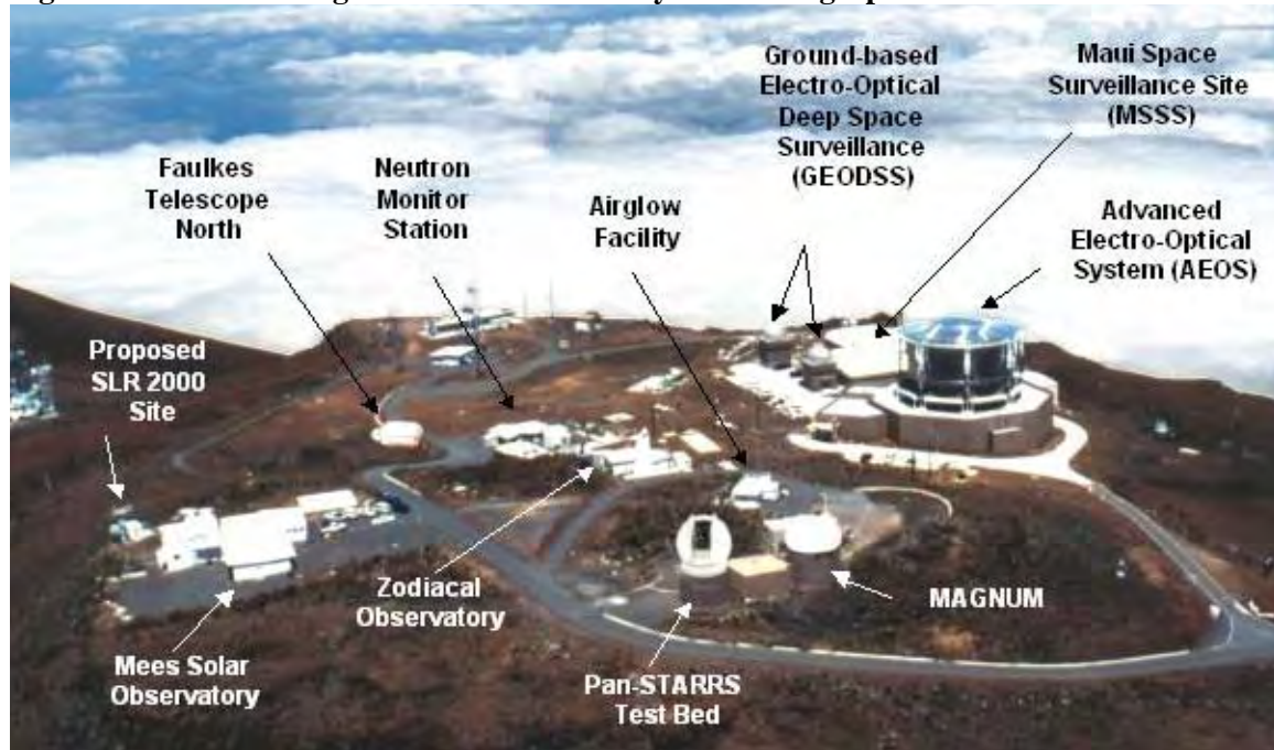
Figure 2. Haleakala High Altitude Observatory Site Photograph
