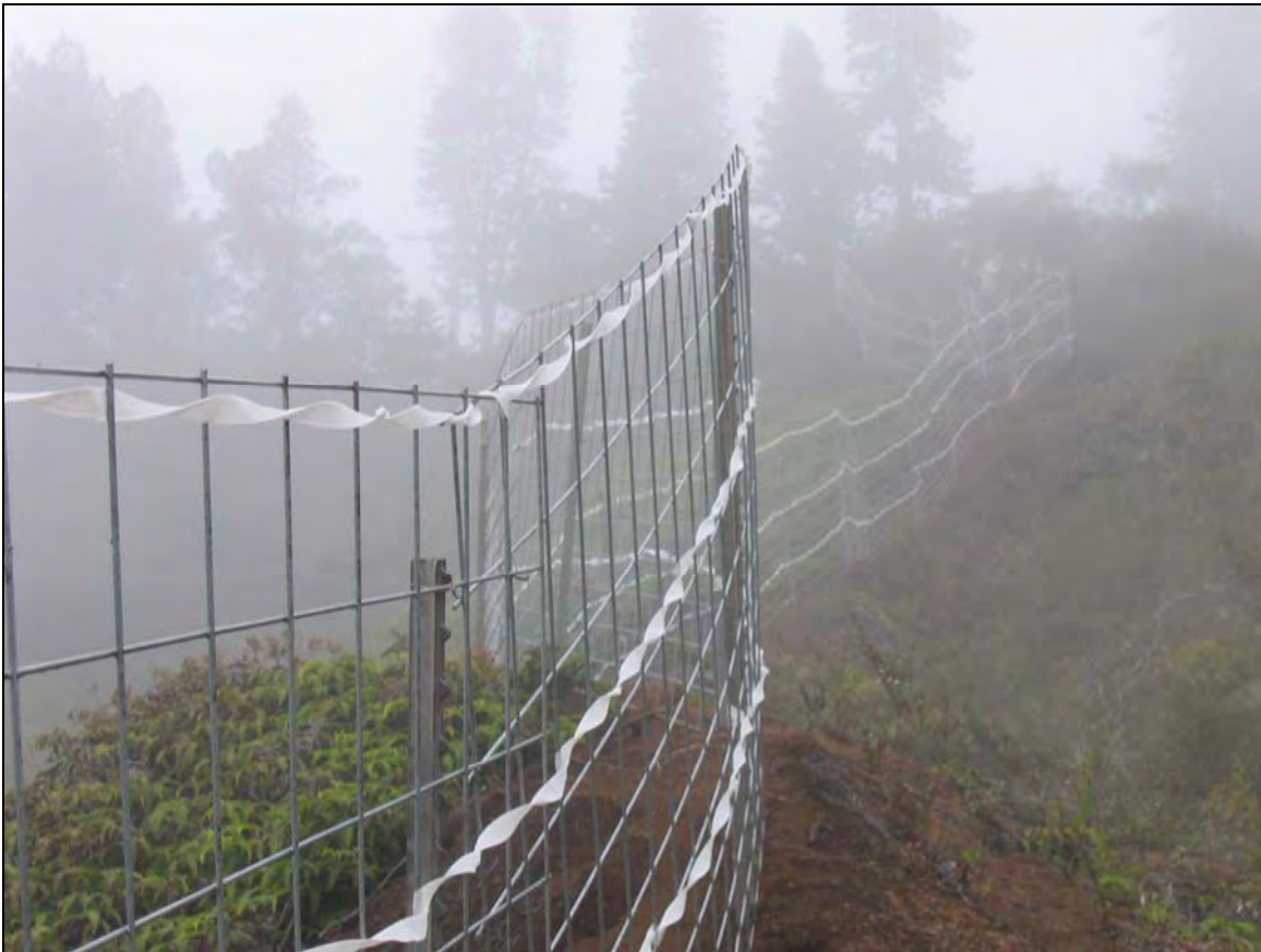
Figure 10. White electric fence polytape improves visibility of lattice structures (Photograph by Jay Penniman, Hawaii Department of Land and Natural Resources, Division of Forestry and Wildlife, 2006).
