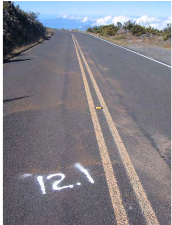
Photo #5 & 6---Segment 2, MP 14.2 & 12.1, Typical pavement distress along centerline of roadway, Note: water flowing through cracks and pavement staining due to migration of fines.
