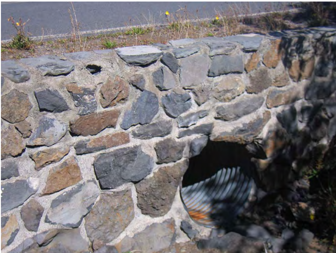
Photo #17-----Typical Metal Culvert with Stone Masonry Hdwls.
