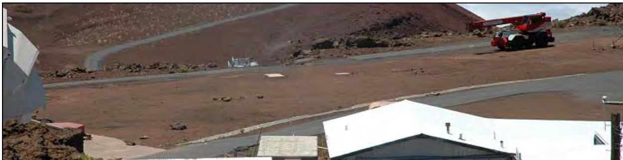
Figure 5. Soil Placement Area A, which will also serve as the equipment staging area - where the truck is parked in this photograph - is a previously disturbed site.
