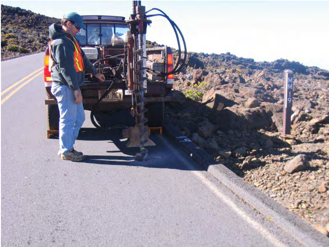
Photo #11---Close-up auguring at MP 19, uphill lane
