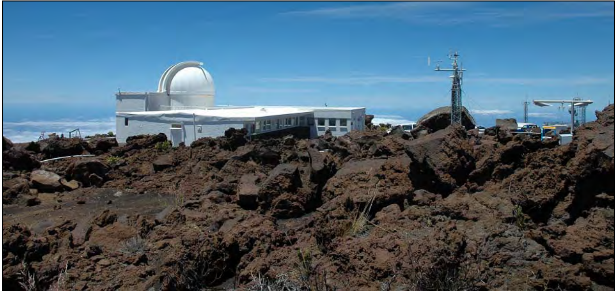
Figure 3. ATST construction site.
