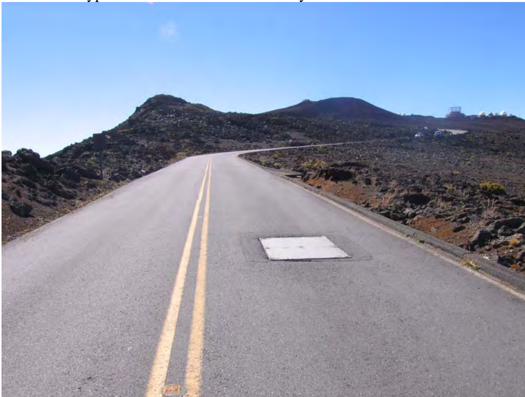
Photo 19 ---MP 20.3, start of under ground utility line in uphill lane, typical bituminous curb shown on the right.
