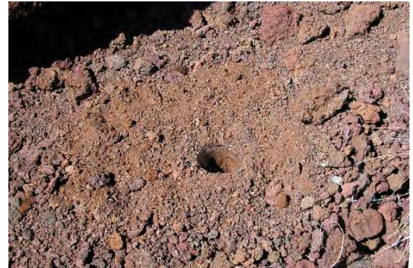
Step 4 Refill hole and create apron
