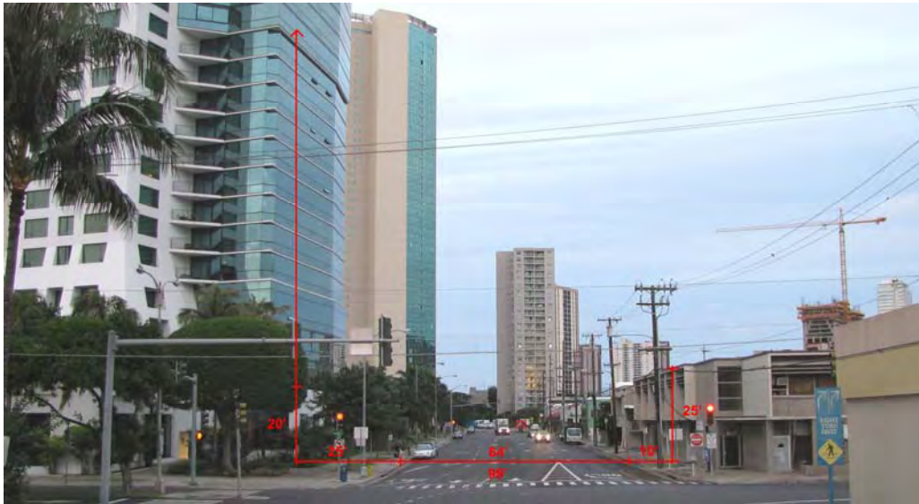
Figure 3-17: Waimanu Street Existing Condition
