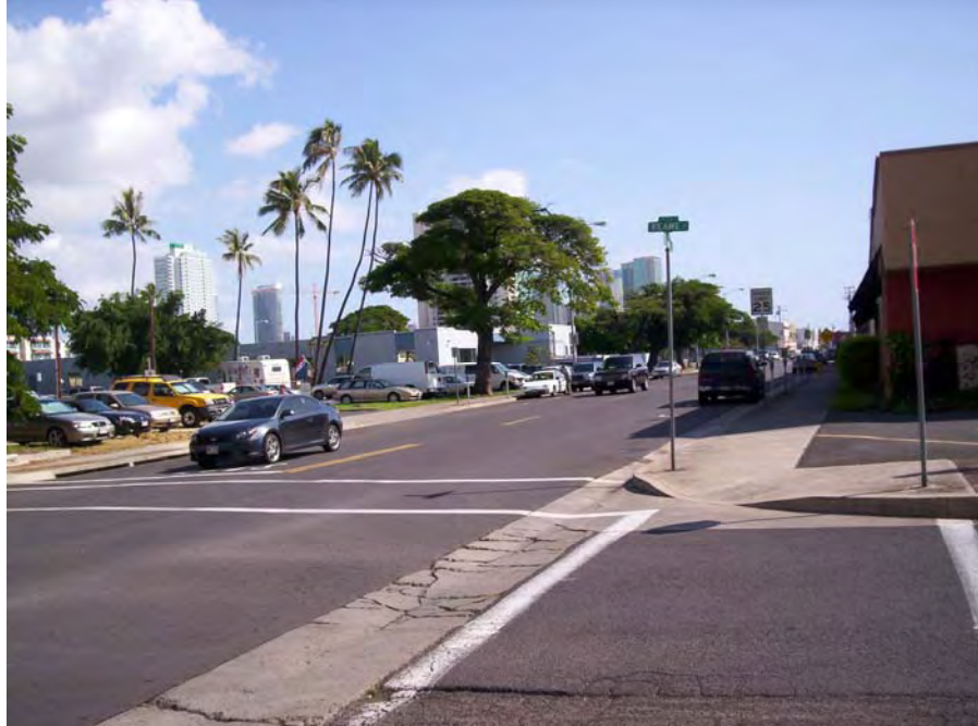
Photo P-3: Intersection of Keawe St. and Pohukaina St. (1/7/08)
