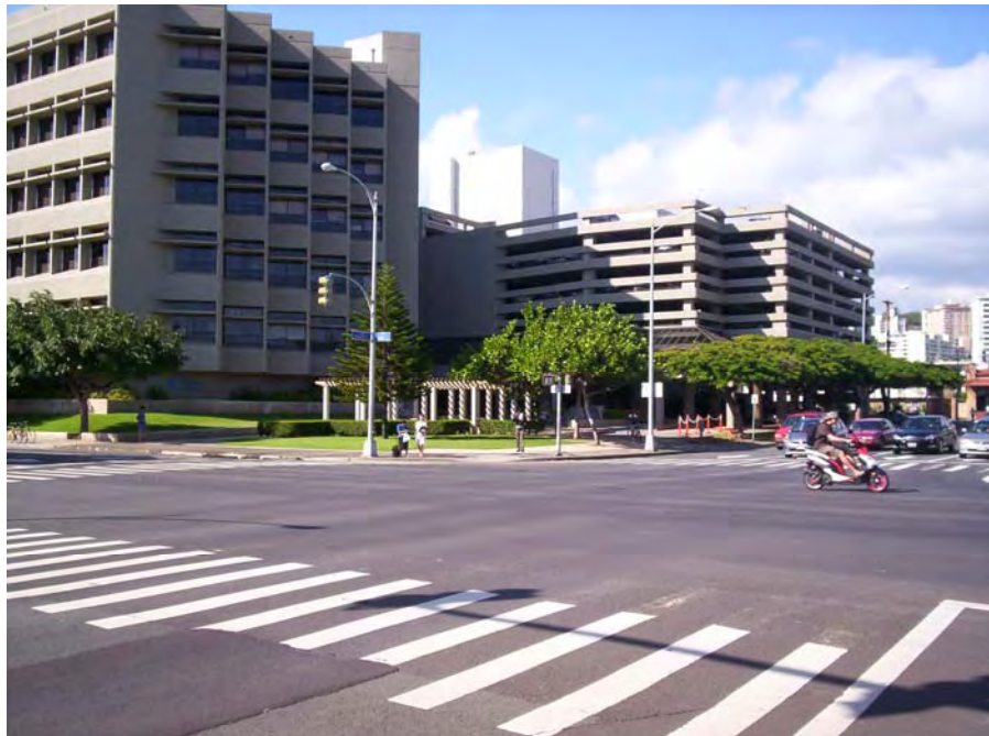
Photo P-20: Intersection of Pensacola St. and King St. (2/19/08)
