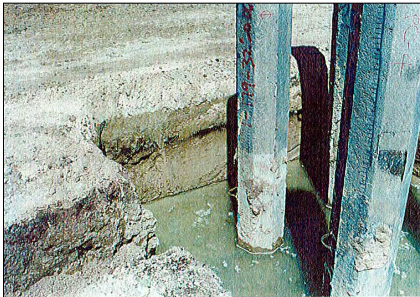
Figure 41. Ward Village Phase II, Ward Theaters, photograph of pile cap trench showing old "A" horizon capping clay pond sediments (Winieski and Hammatt 2001)
