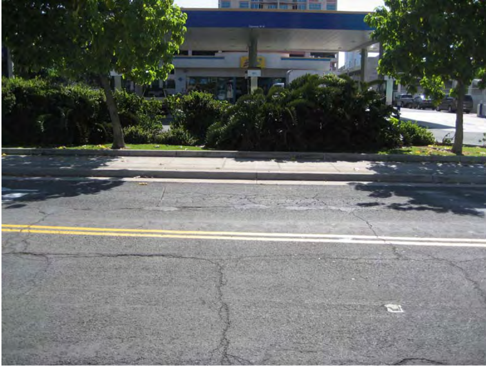
Photo P-5: Cooke Street Alligator & Block Cracking
