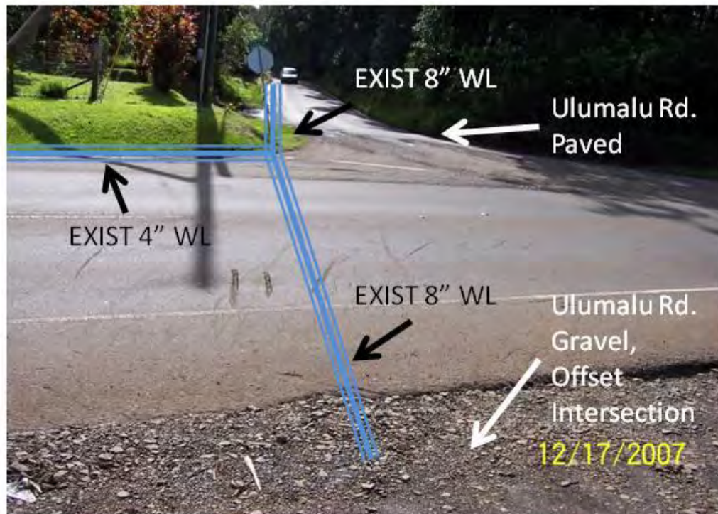
PHOTO 1 = ULUMALU ROAD AND HANA HWY. INTERSECTION. LOCATION OF EXISTING DEPARTMENT OF WATER SUPPLY WATERMAIN STUBB-OUT FOR PROPOSED WATERLINE
