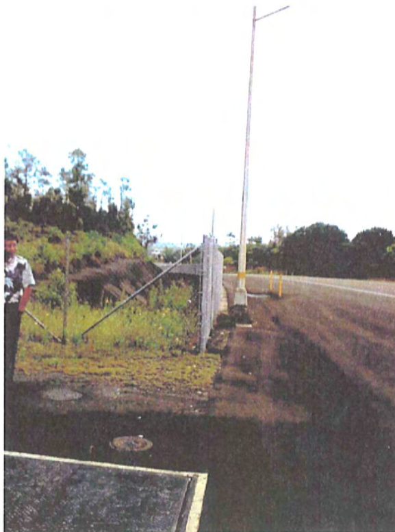
Existing Utility Laterals fronting the Proposed Site (10/18/07)
