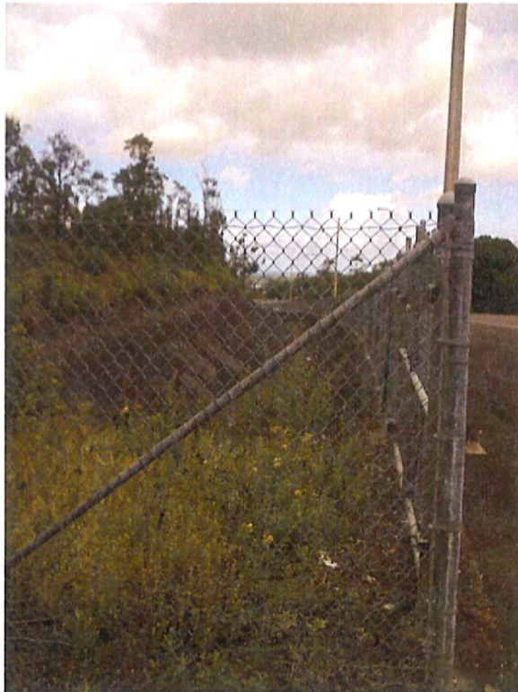
Fence Around County Lined Open Ditch along Mohouli Street (10/18/07)
