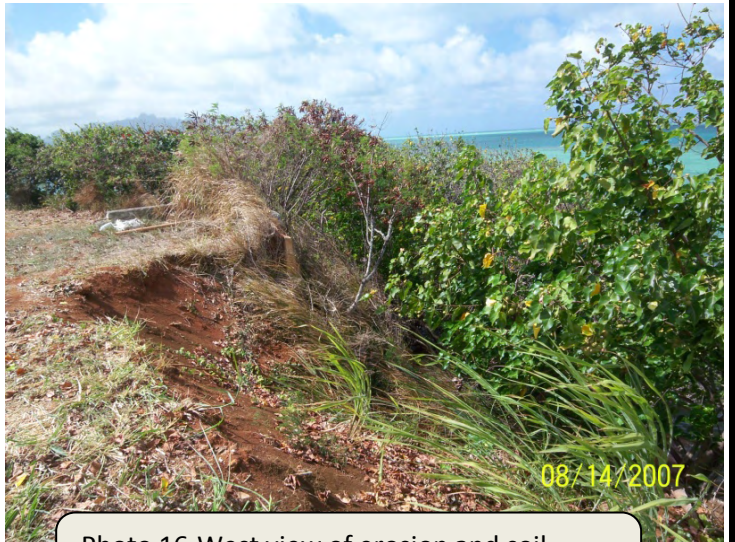
Photo 16-West view of erosion and soil slippage at top of bank.
