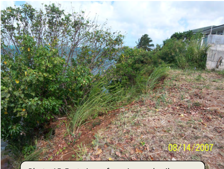
Photo 15-East view of erosion and soil slippage at top of bank.
